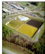
Figure 1. Photograph of the S-3 waste ponds before capping, at the Field Research Center (FRC) site of the U.S. Dept. Of Energy Environmental Remediation Science Program at Oak Ridge, TN. These ponds received a mixture of nitric acid, organic solvents, uranium, technetium and other heavy metals at rate of approximately 10 6 L of waste per year for 30 years before their closure in 1984.
