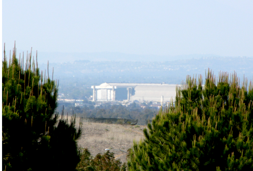
Figure 13 A view of Tustin Air Force Base hangars from the Irvine hills (photo by author)
