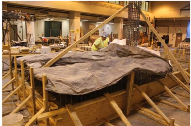
Figure C.7 Finishing the concrete surface after first lift (left); and covering the deck slab fresh concrete with curing blankets to avoid shrinkage cracks (right)
