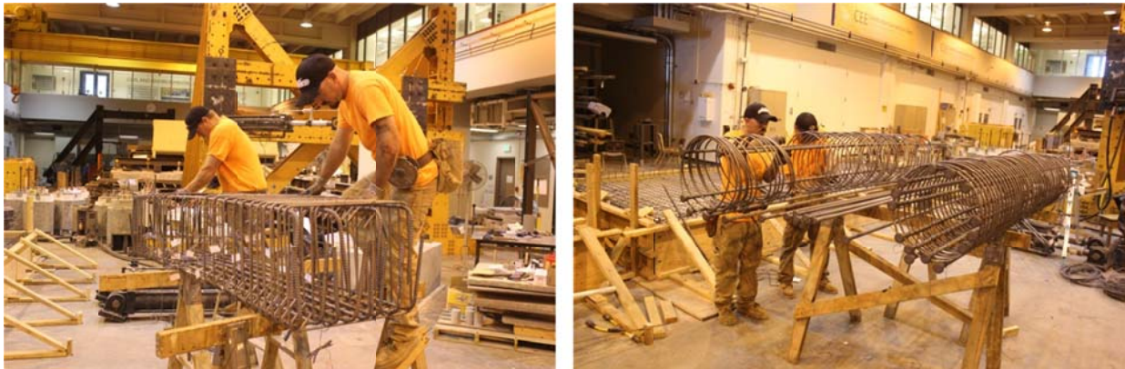
Figure C.4 Fabrication of the bent cap beam (left) and columns (right) cages
