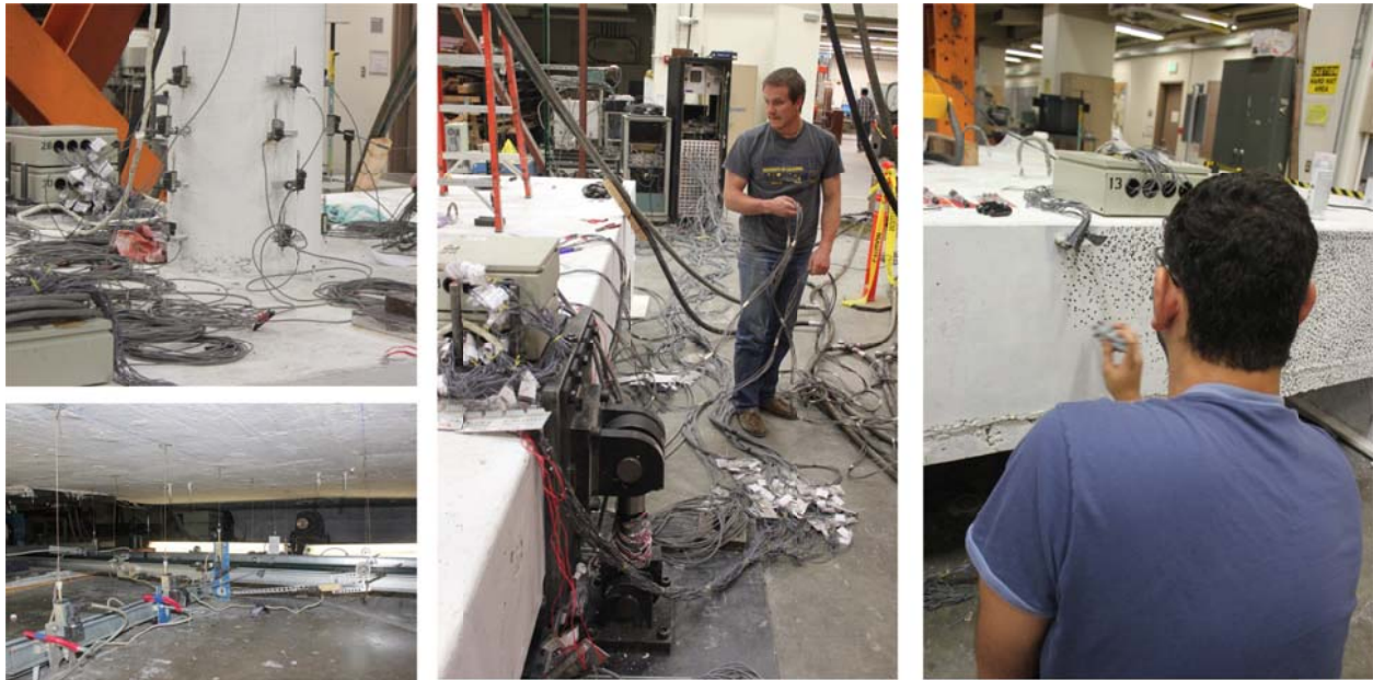
Figure D.10 Different stages of instrumenting the test specimen with LVDTs at the column expected plastic hinge zone (top left), and under the specimen (bottom left); extending instrumentation cables (middle); and preparing the specimen for digital image correlation advanced monitoring technique (right)
