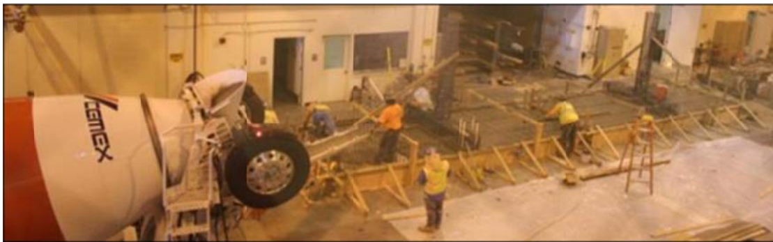
Figure 3.18 Seat beams and box-girder deck slab concrete placement (first lift)
