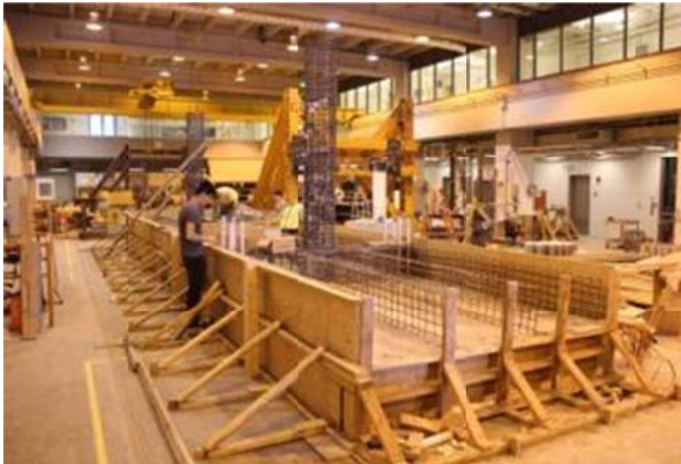
Figure C.8 Setting up the side formwork for the second construction phase to build the box-girder (left); and installing special custom-made cardboard boxes for the box-section cells (right)
