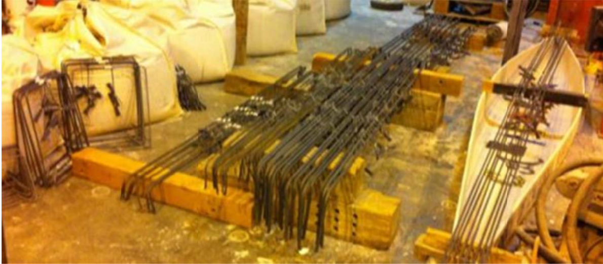
Figure 3.42 Instrumented specimens' beam and slab reinforcement bars
