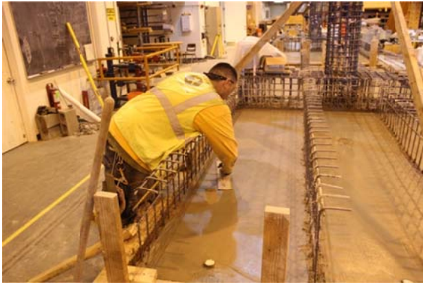
Figure C.7 Finishing the concrete surface after first lift (left); and covering the deck slab fresh concrete with curing blankets to avoid shrinkage cracks (right)
