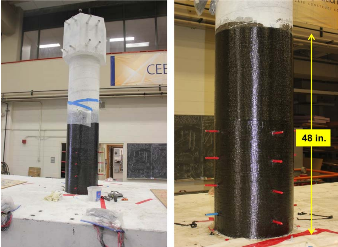
Figure 8.5 An overview (left) and close-up view (right) of the final retrofitted column of SP2
