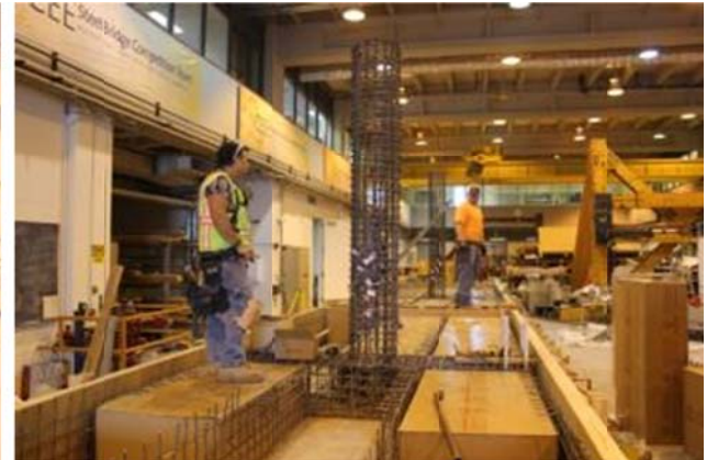
Figure C.8 Setting up the side formwork for the second construction phase to build the box-girder (left); and installing special custom-made cardboard boxes for the box-section cells (right)
