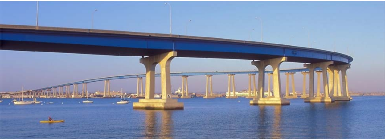
Figure 1.1 San Diego- Coronado box-girder bridge, California (Photo: Brett Shoaf, Artistic Visuals)
