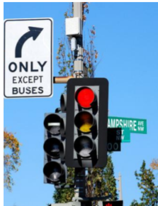
Bus queue jump signal next to traffic signal (Photo: BeyondDC via Flickr, CC BY 2.0)
