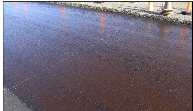
Figure 3.6: Close-up view of tack coat application.
