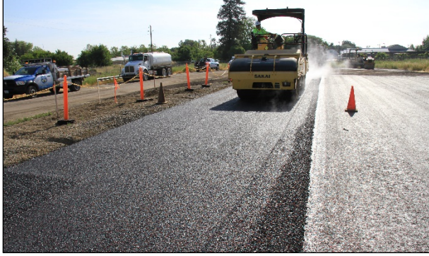
Figure 3.10: Breakdown compaction (Section J).
