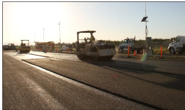
Figure 3.12: Final compaction (Sections H and I).
