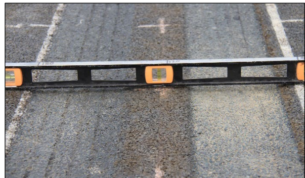
Figure 5.41: 701HC: Close-up view of test section surface at Station 8.
