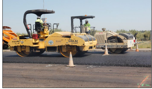
Figure 3.11: Breakdown (Section G, front) and intermediate compaction (Section J).
