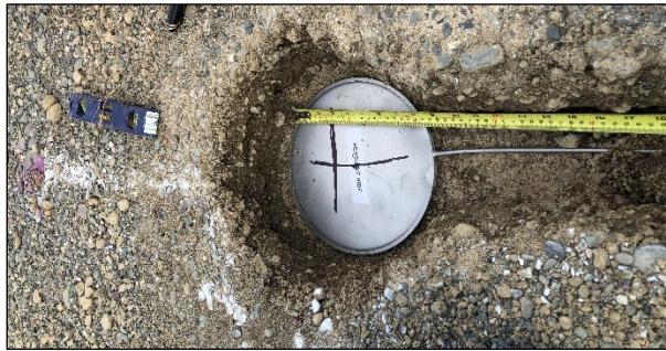
Figure 4.3: Pressure cell installation.
