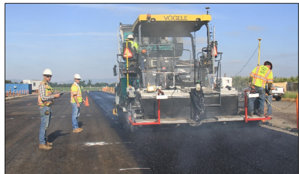
Figure 3.9: Paving first lift of RHMA-G (Section J).
