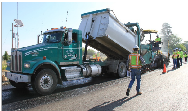
Figure 3.8: Dumping mix into the paver (Section J).
