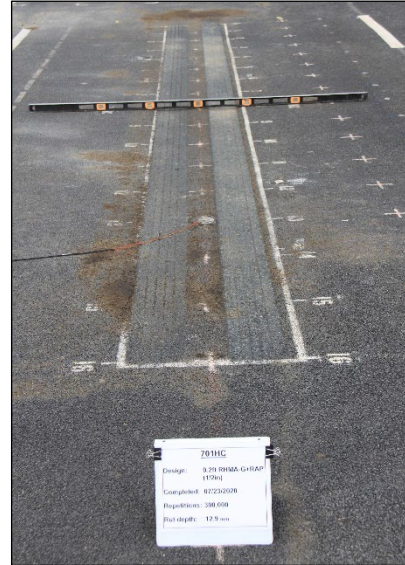
Figure 5.39: 701HC: Test section view from Station 16.
