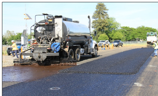
Figure 3.7: Tack coat application between lifts of RHMA-G (Section J).
