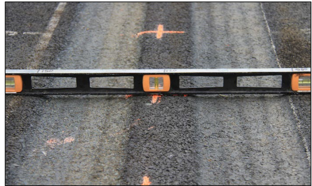
Figure 5.20: 704HB: Close-up view of surface at Station 8.
