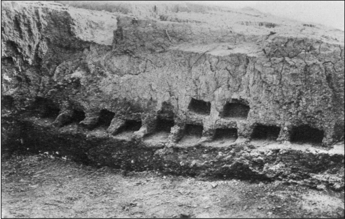
FIGURE 217. Room 15, with two tiers of pigeonholes across its southwestern end, House of Nabu, Khorsabad. Loud and Altman 1938: pl. 24 D.
