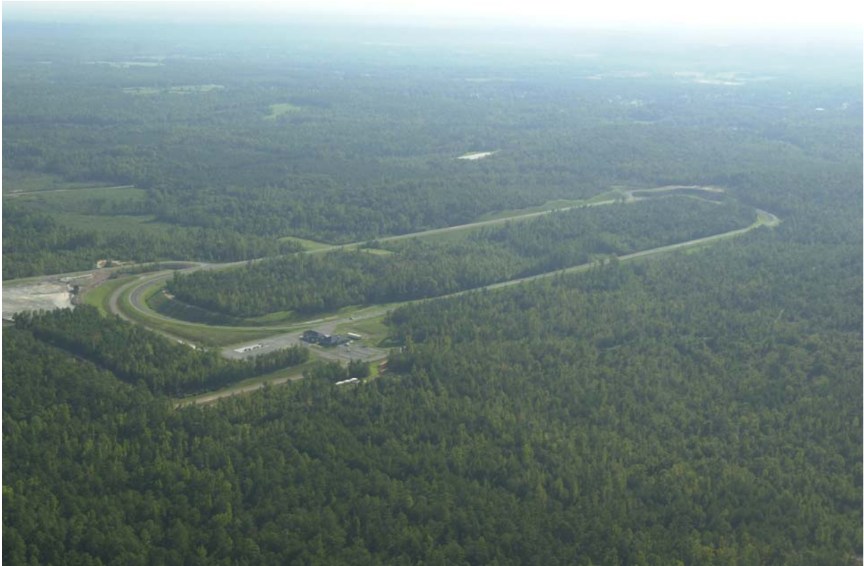
Figure 2.1: Overview of the NCAT track facility. (Taken from the photo album on the NCAT website: www.pavetrack.com/images/photo%20album/ ).
