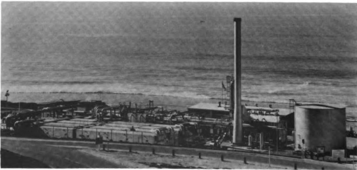
Figure 4-50 A multistage flash seawater desalination plant with a capacity of 3800 m 3 /day, originally located at Point Loma, California, and subsequently transferred to the United States Guantanamo Naval Base in Cuba. ( The Fluor Corp., Ltd., Los Angeles, Calif. )
