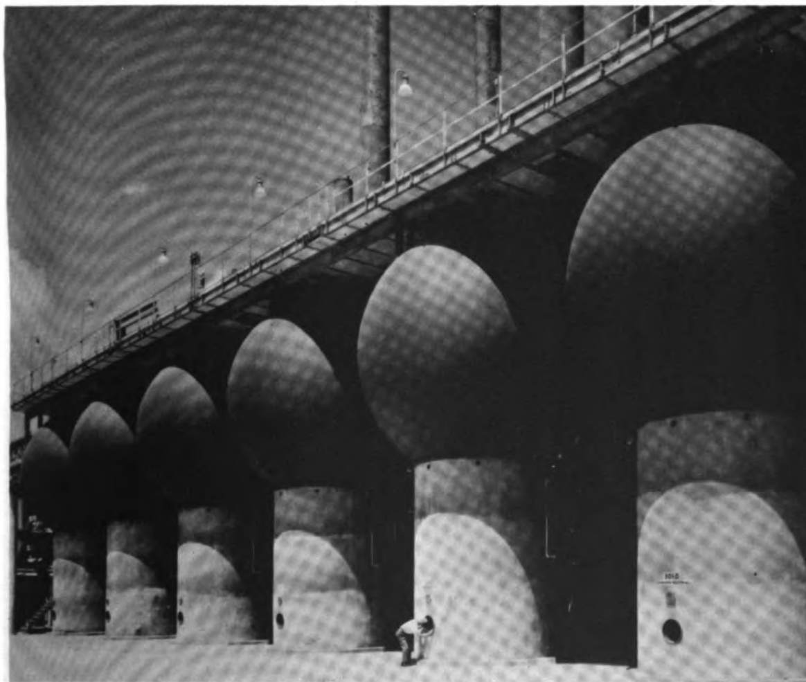
Figure 1-9 Six spheroidal reactors in a catalytic reforming unit at the Texas City, Texas, refinery of the American Oil Company. (Pullman Kellogg Co.)
