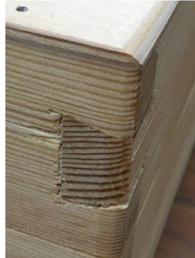
Figure 4: Dovetail joint constructed by professional.
