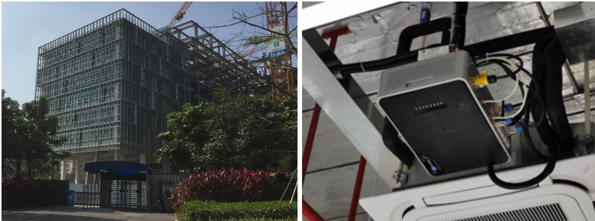
Figure 6: The eight-floor IBR DC office building, still under construction (left). IBR's power distribution box for 48 V distribution over each floor (right).
