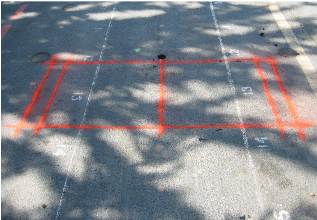
Figure 3.34: Section surface between Stations 12 and 15 at end of test.
