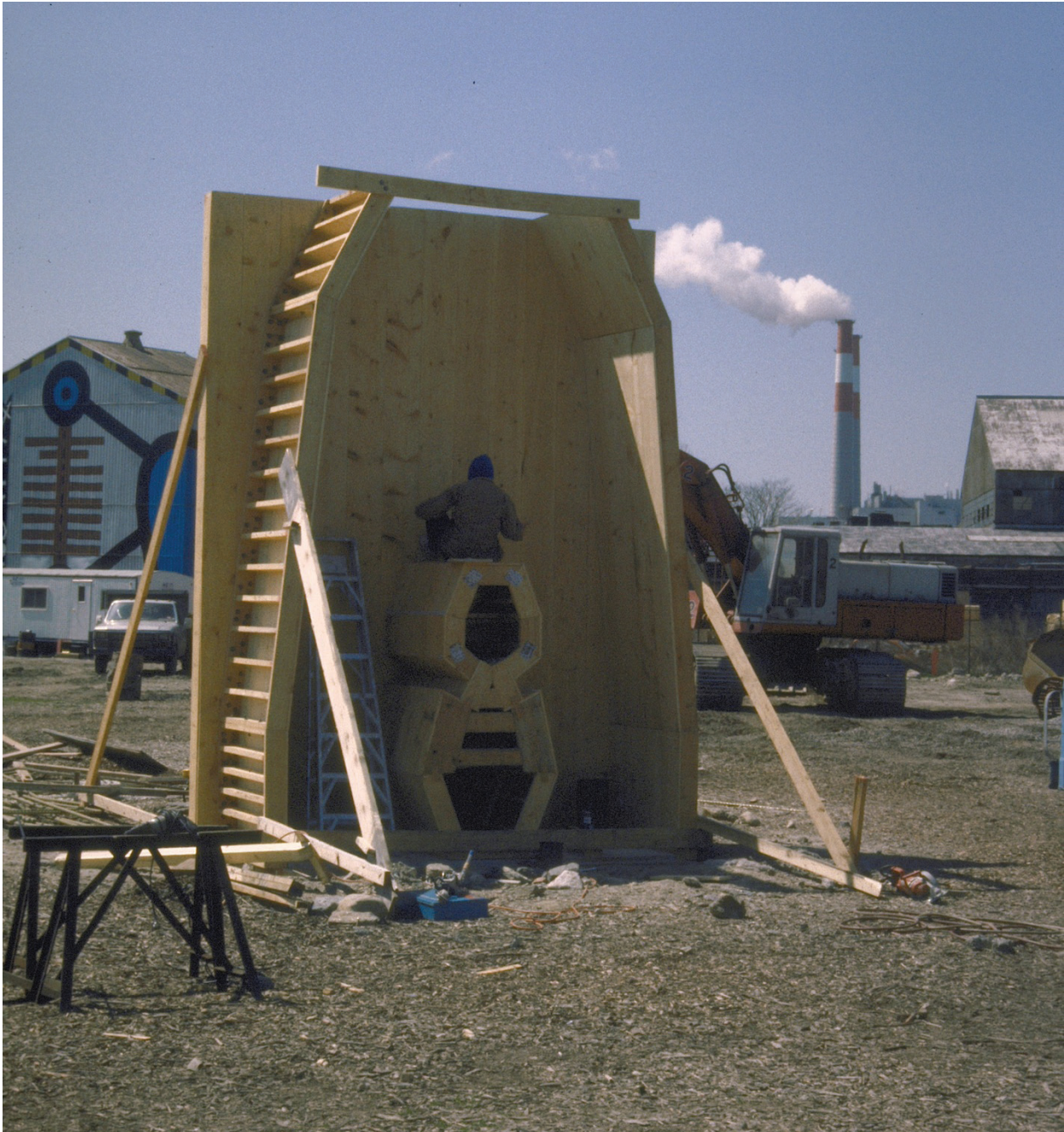
Formwork for Cast Concrete, 1990, Socrates Sculpture Park, 16 x 10 x 4 feet
