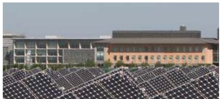
UC Merced installed a 1-megawatt solar array to help meet zero net energy on campus.
