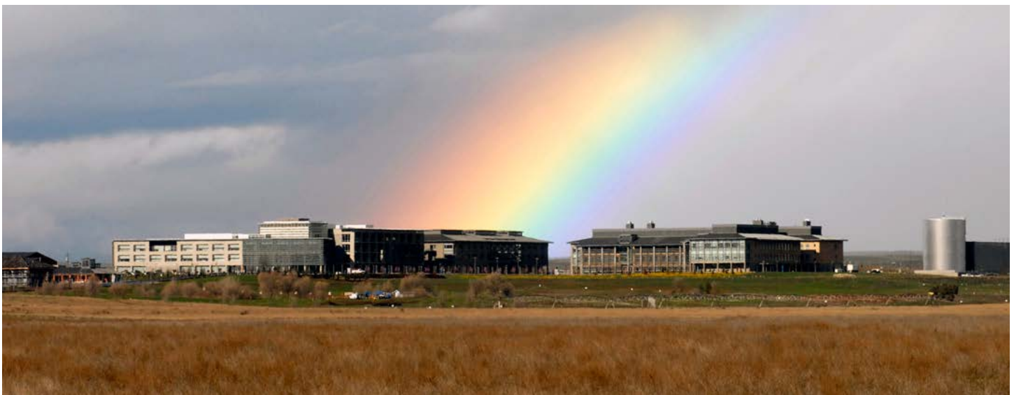
A rainbow touches down over the UC Merced campus. The Central Plant can be seen on the far right; the Science & Engineering building is directly to the left of the plant.
