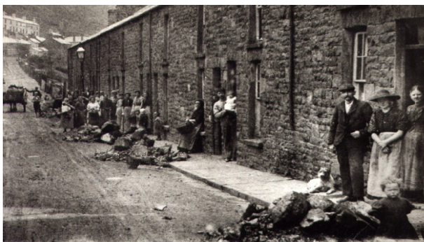
Fig. 2 Poor housing conditions in Rhondda (1920-1970).
