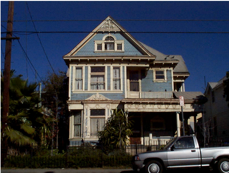
Figure 6.78: Example of Queen Anne style home in the University Park HPOZ. Source: (Office of Historic Resources n.d.).
