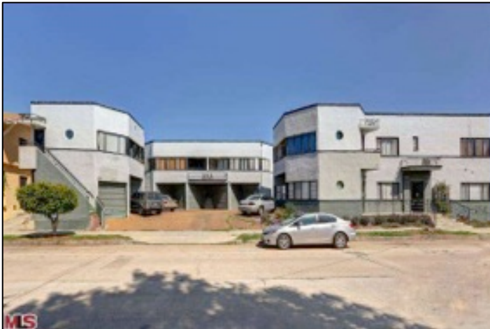
Figure 6.9: 1000 West Edgeware Road. 7 units. Built 1931. Streamline Moderne. Source: Redfin.com
