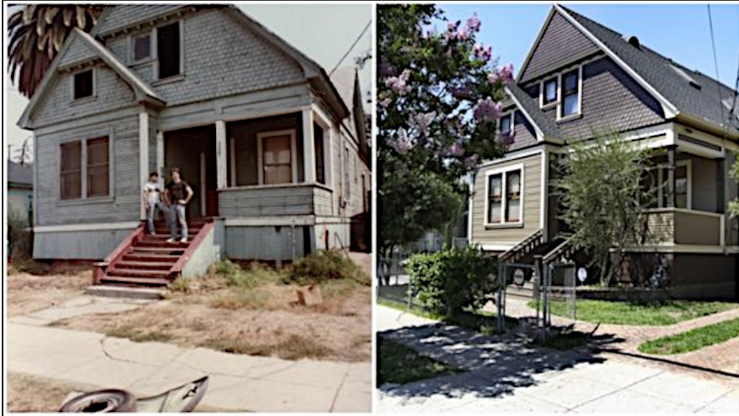
Figure 6.21: Restoration at Bellevue Avenue. Before: Danny Muñoz and David Hiovich (left) stand in front of their home in 1981. After: The same house today (right). Photos by Jesse Saucedo. Source: (Lion 2012).
