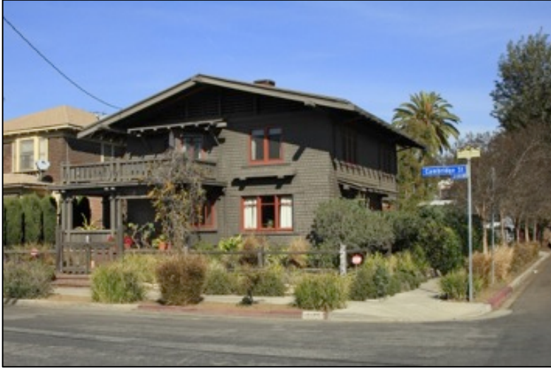
Figure 6.60: The Lucy Wheeler house, built in 1905, is the last remaining Greene and Greene house in the city of Los Angeles. It is a Historical Cultural Monument. Source: Los Angeles Office of Historic Resources.
