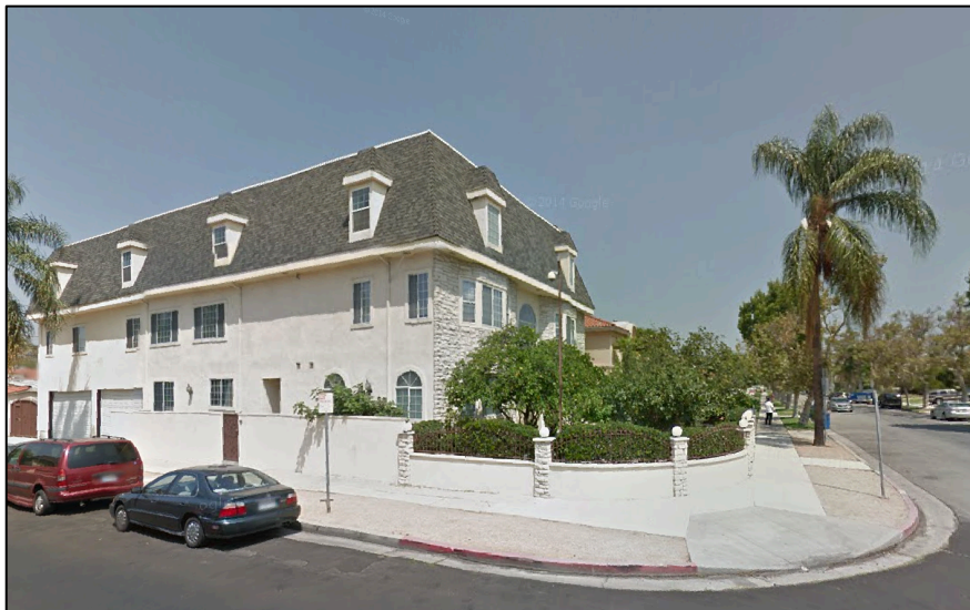
Figure 6.53: The property at the Northwest corner of Poinsettia and 2 nd Street in Miracle Mile North. Image: Google Street View.
