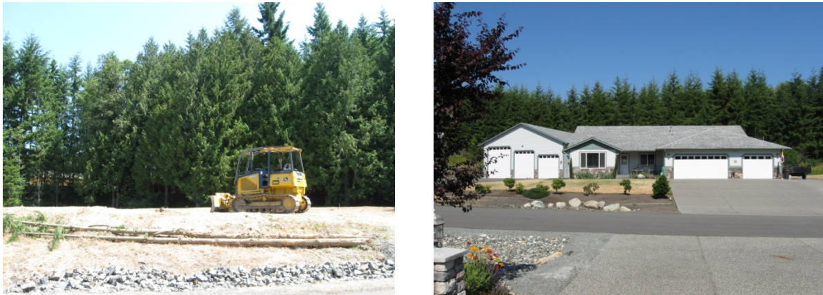
Figure 1 Examples of 1 acre residential lots in Snohomish County immediately following site clearing and post-construction
