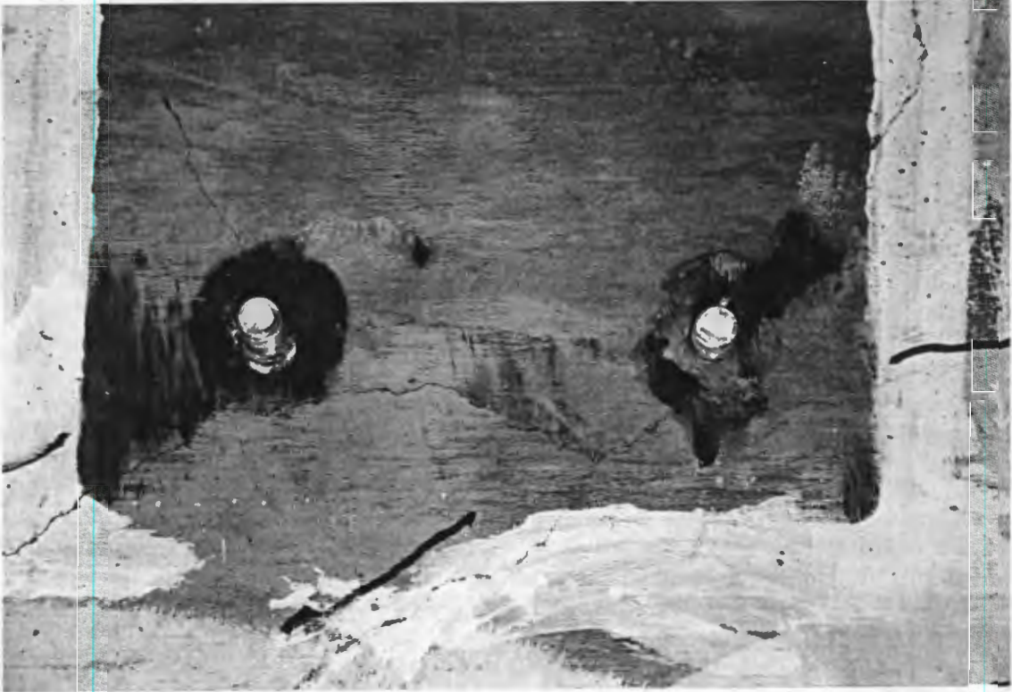
Figure 7.21. Close-up of the epoxy around the studs after the last test
