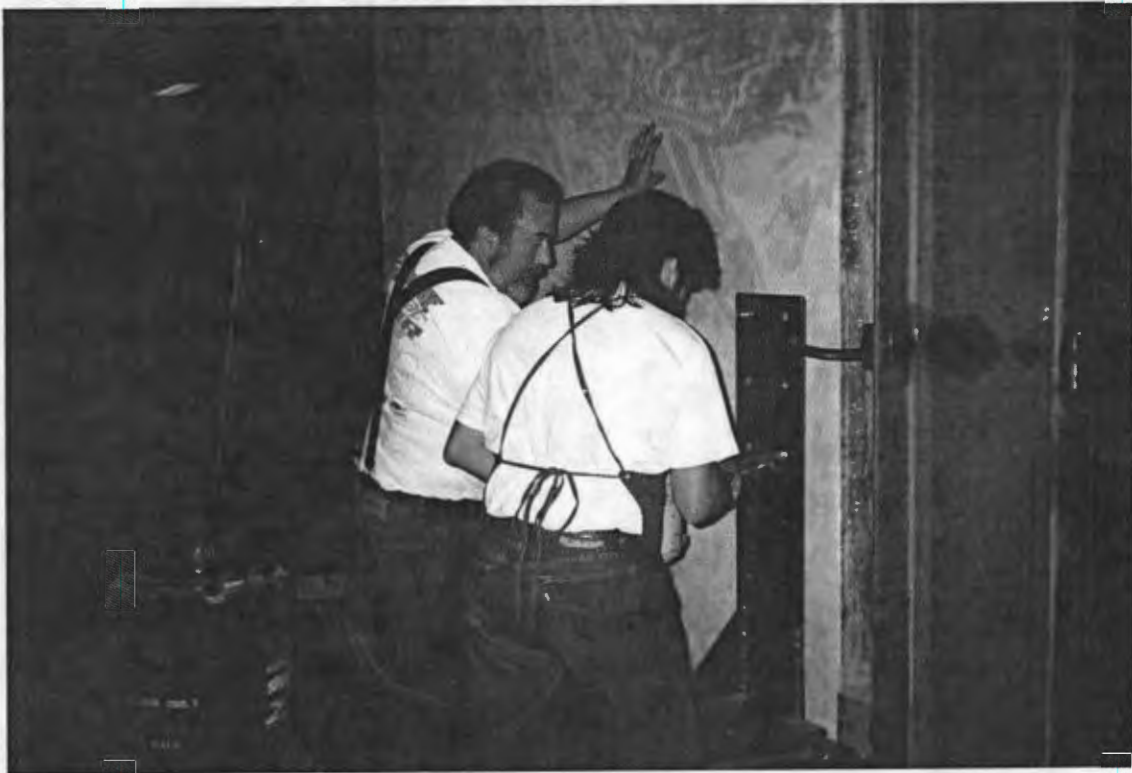
Figure 5.1. (a) Hilti Kwik Anchor Bolt, (b) Bolt installation at the bottom support
