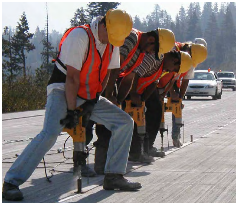
Figure 5. 2 Magnet Installation
