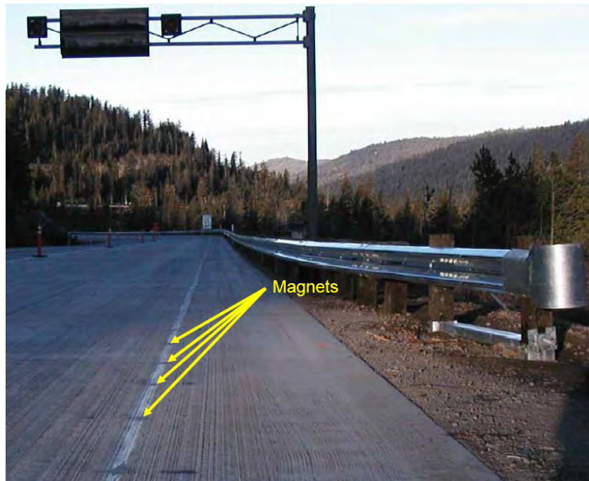
Figure 5. 3 Magnets along guardrail
