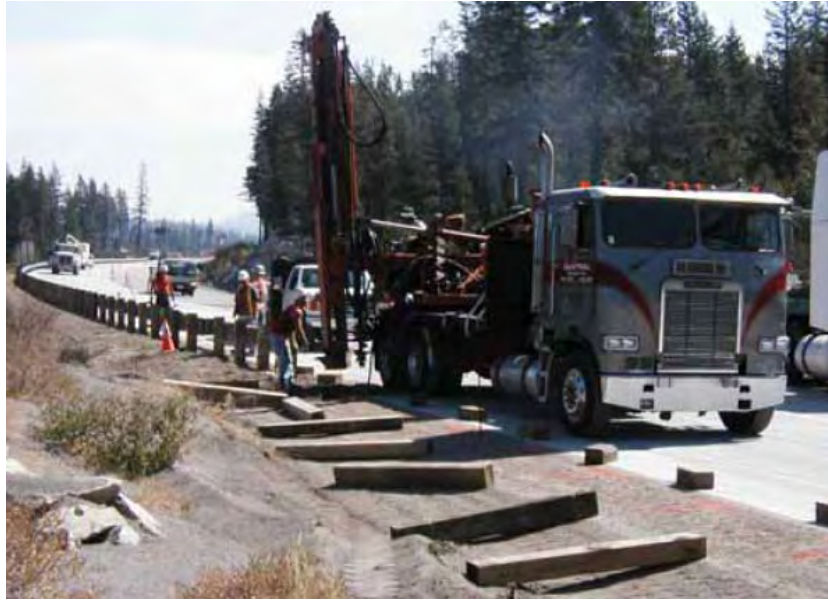
Figure 1. 3 Example of guardrail rehabilitation
