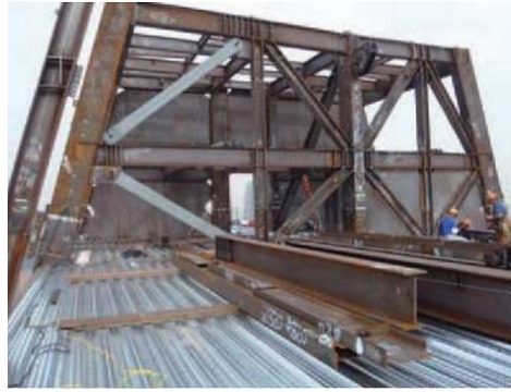
Installation of buckling-restrained braces in the roof
