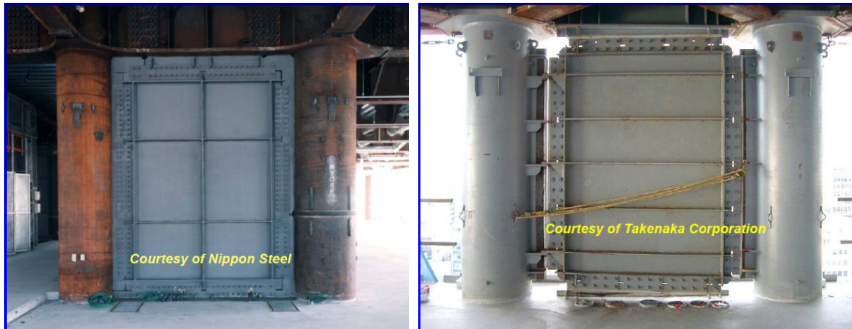
Figure 1.2 Examples of stiffened steel shear walls used in Japan (Photo courtesy of Nippon Steel and Takenaka Corporation)
