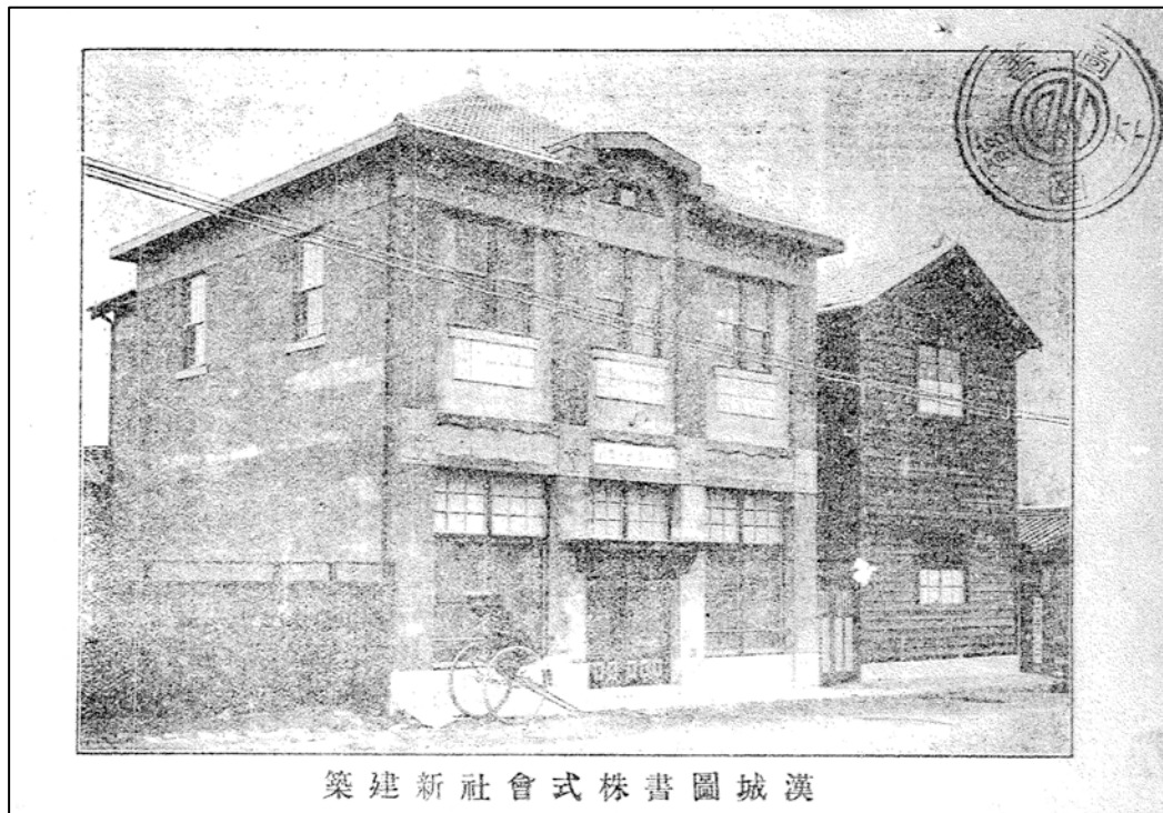
Figure 1. The newly built Hansŏng Tosŏ Chusik Hoesa Building. Source: Haksŏnggye (December 1920, unnumbered front matter). Image from microfilm at the National Library of South Korea.
