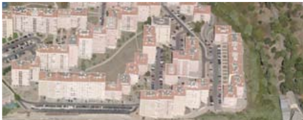
High density housing illustrates typical new construction.
