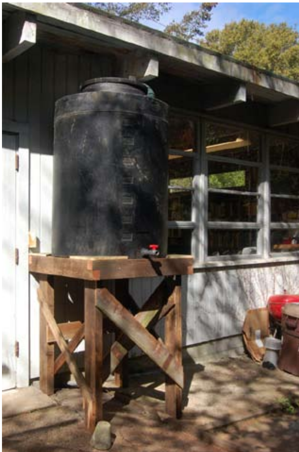
A cistern catches rainwater from the roof which is then used to irrigate the surrounding landscape plantings.
