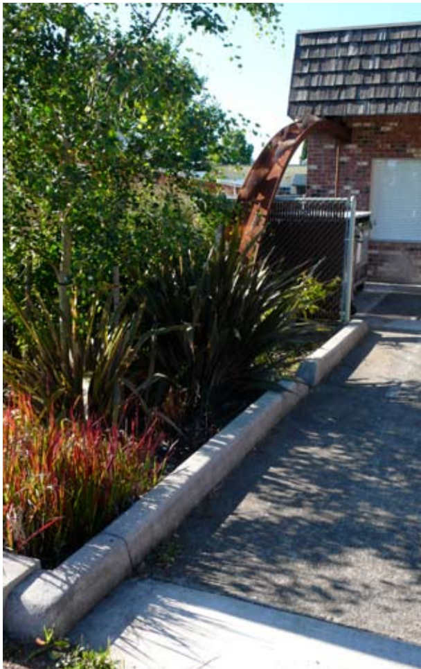
A raingarden in Portland, Oregon accepts runoff from the roof of the adjacent building.
