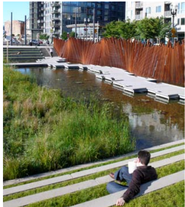
A constructed stormwater wetland also functions as a park in downtown Portland, Oregon.
