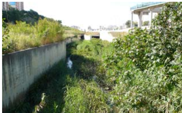
Ribeira dos Ossos at the culvert of Ribeira das Jardass
