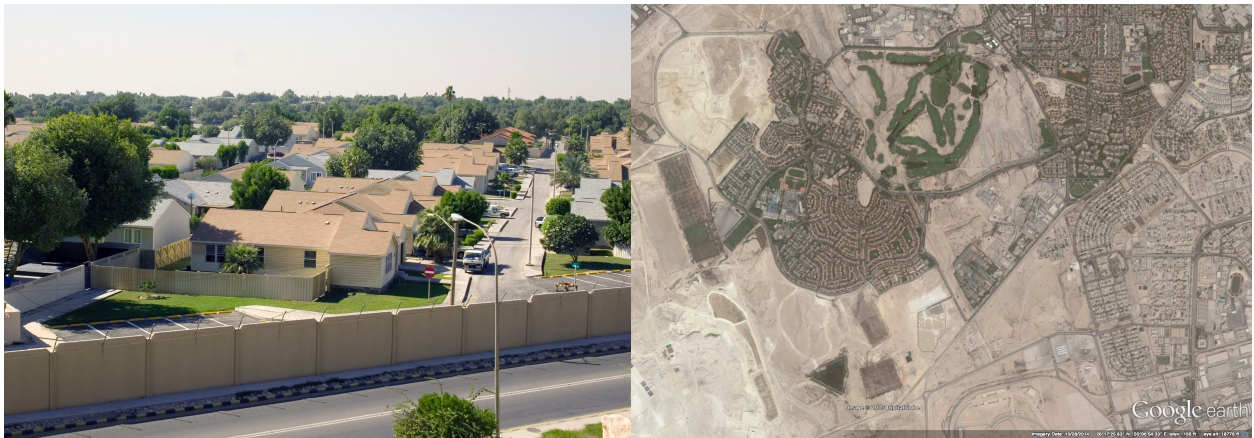
Figure 2 (left): Aramco Dhahran Compound showing typical suburban pitched roof houses. The wall fence is visible in the foreground.
