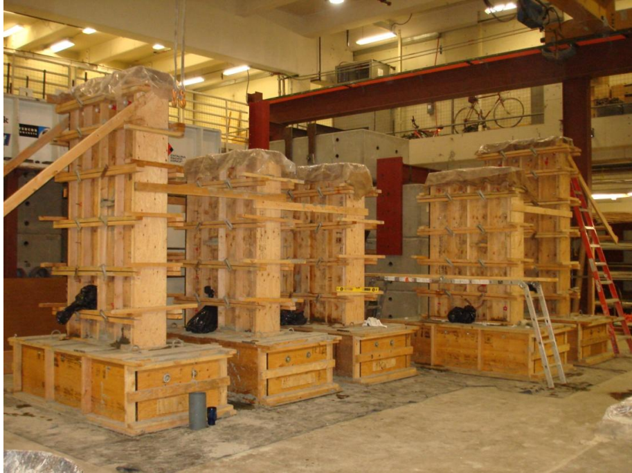
Figure 5-15 Formwork and shoring for specimens
