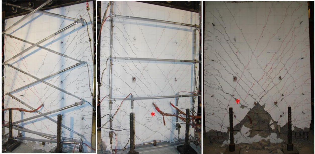
Figure 6-14 RW-A15-P10-S51: Crack patterns at drifts of 0.5%, 1.5%, and at end of test
