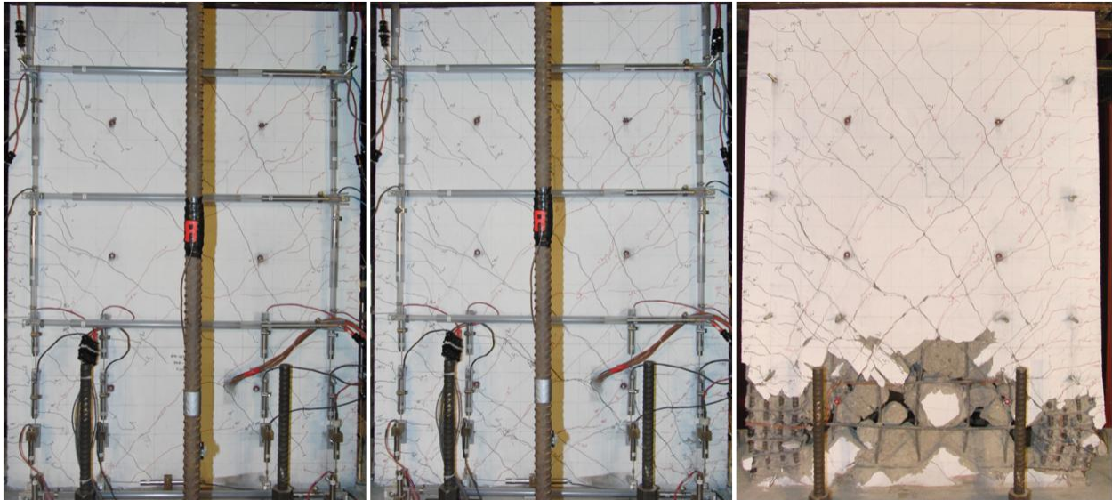
Figure 6-28 RW-A15-P2.5-S64: Crack patterns at drifts of 0.5%, 1.5%, and at end of test
