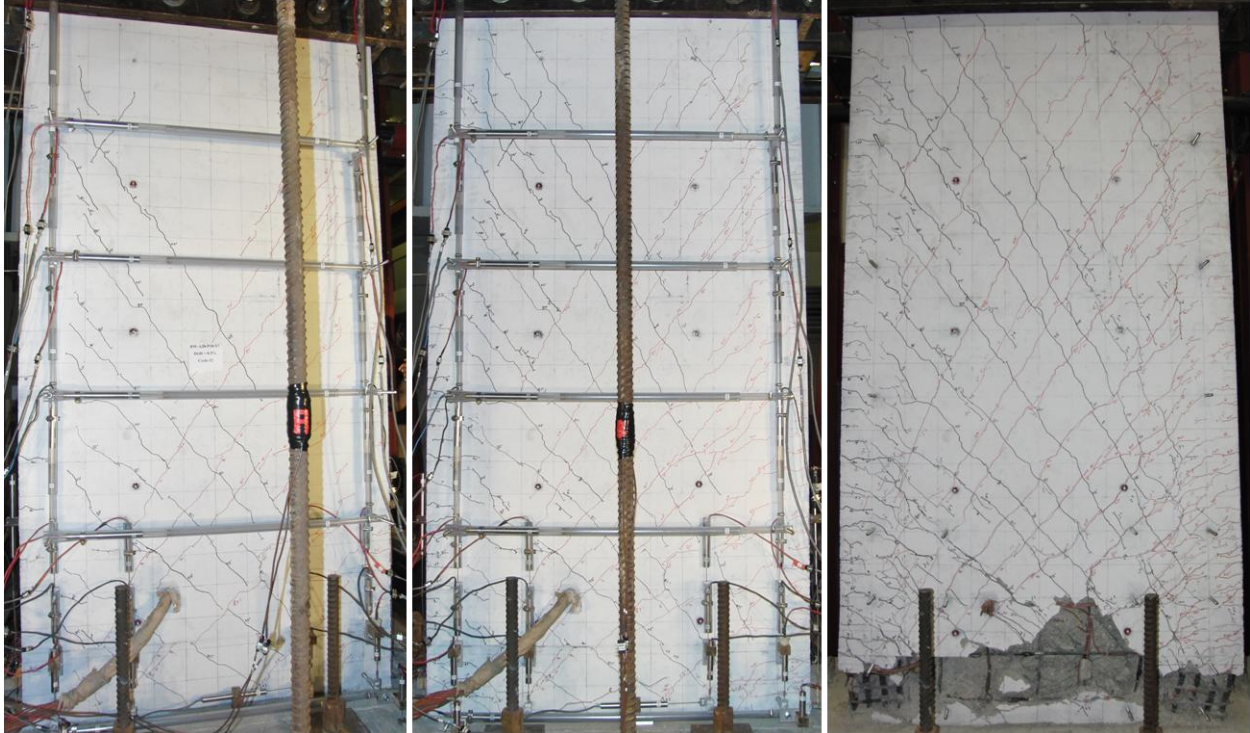
Figure 6-8 RW-A20-P10-S63: Crack patterns at drifts of 0.5%, 1.5%, and at end of test
