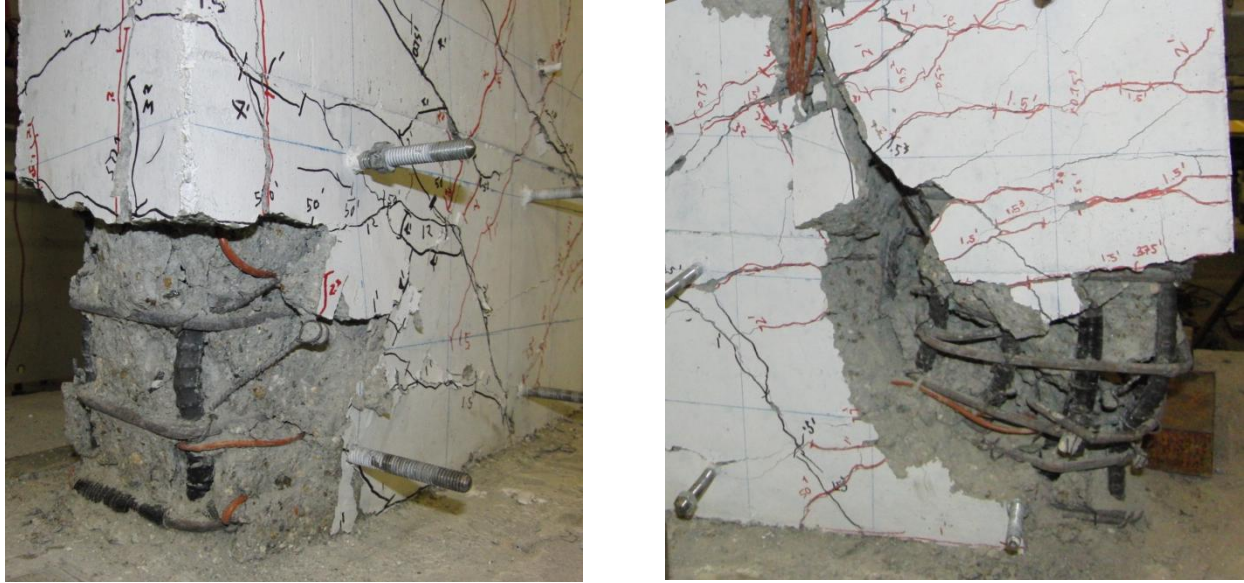
Figure 6-7 RW-A20-P10-S38: North and south wall boundaries at end of test
