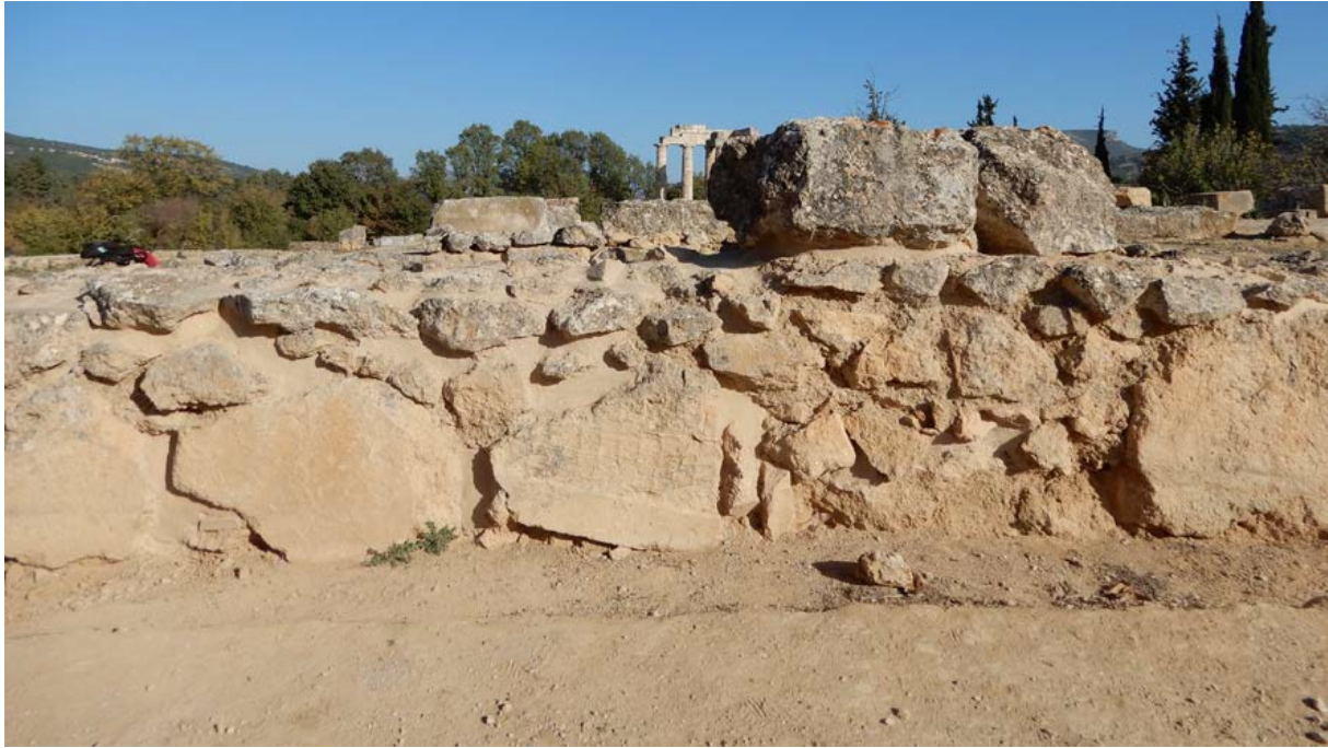
Figure 2. Basilica, S façade, post conservation
