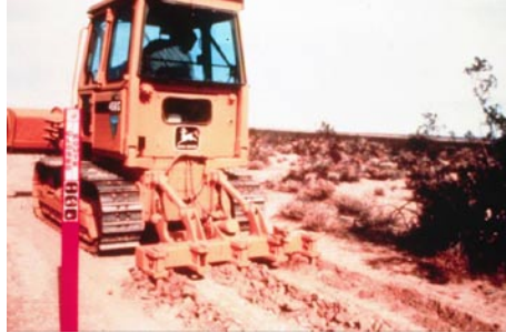
Fig. 1. Ripping the roadbed. (Photo: Daniel Patterson)
