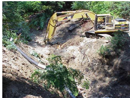
Fig. 3. Full road recontour, Clearwater National Forest, ID. (Photo: Bethanie Walder)
