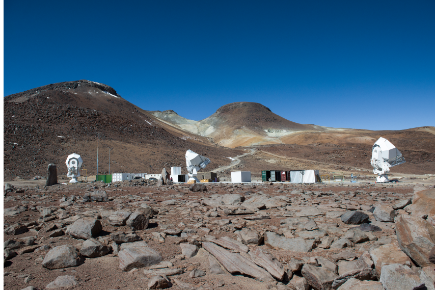
Figure 2.13: Photo of the three telescopes that comprise the Simons Array. The left telescope houses the POLARBEAR-2a receiver and is currently operable. The right telescope will soon house the POLARBEAR-2b receiver, while the center telescope is the original HTT housing the POLARBEAR-1 receiver and will eventually be retrofitted for the POLARBEAR-2c receiver. Photo courtesy of Praween Siritanasak.
