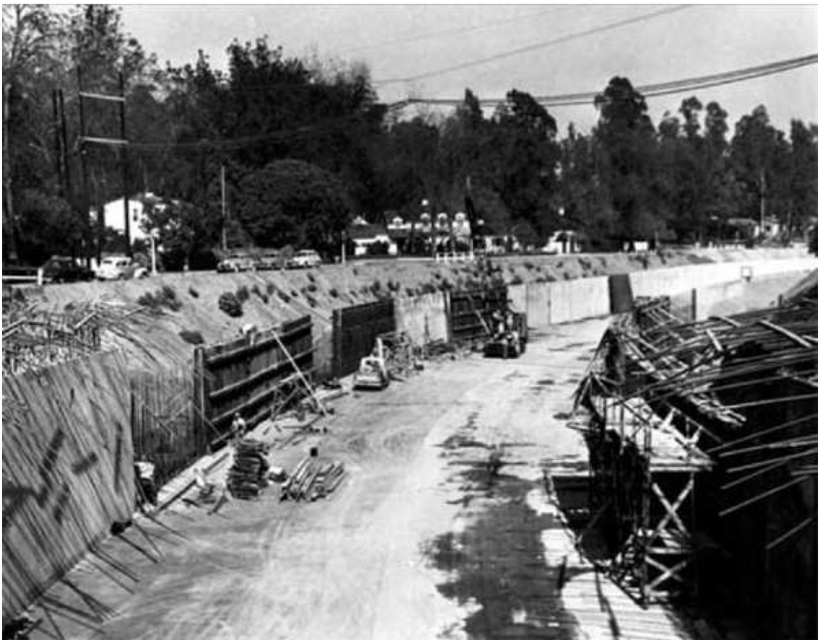
Figure 3.2 Containing of the Los Angeles River c.1930
