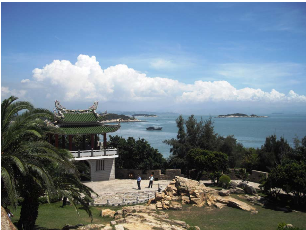
Figure 24. The island of Tongshan, present-day Dongshan, served as a subsidiary base of the Zheng organization. The walls, partly shown here, and the main fortress were built during the sixteenth century to repel piratical attacks. Photograph by author, 2009
