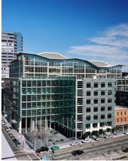
Figure 11: 405 Howard St. Building
