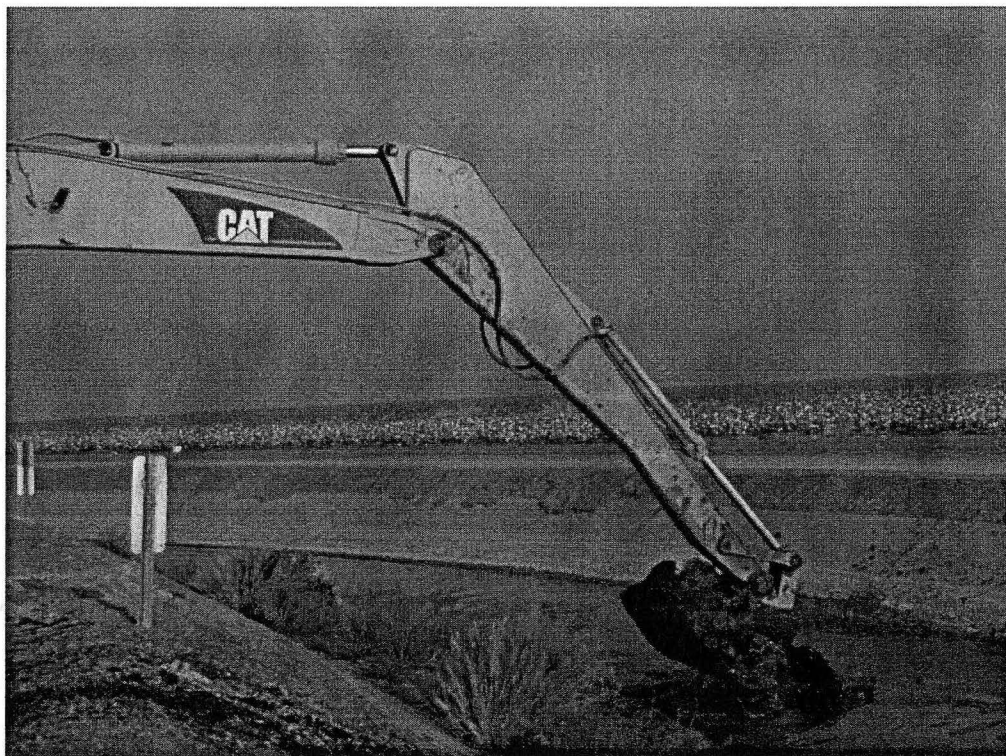
Figure C.4. Dredging of SLD sediment.
