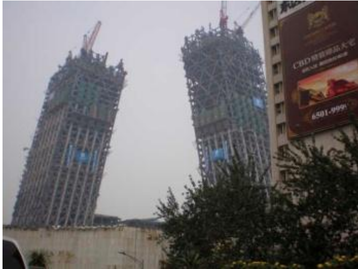
Figure 0.2. Rem's half-built CCTV tower in Beijing in 2004
