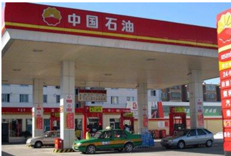
Figure 5.10. Gas station as landmark. Source: Image by Tycho de Feyter on his blog (de Feyter 2012)
