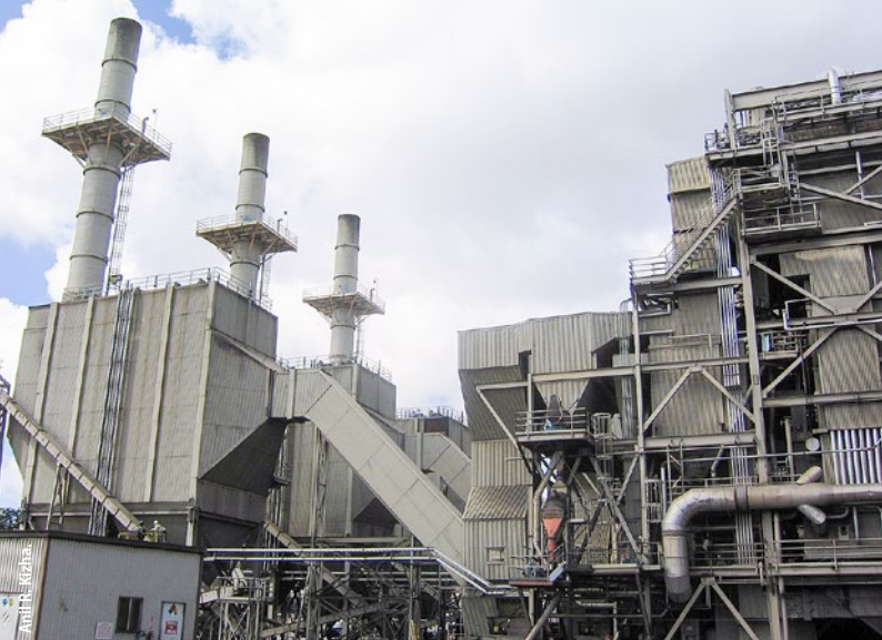
Blue Lake Power in Humboldt County, which utilizes 87,500 BDT per year to generate 10 MW of electricity, receives most of its biomass from sawmills.
