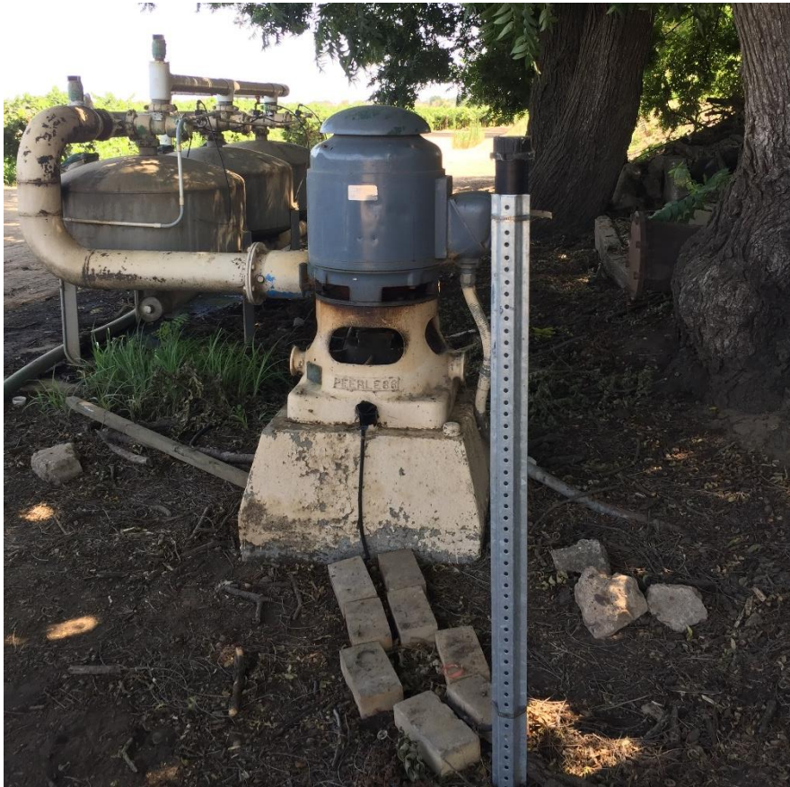
Figure A2. Installation of a telemetry unit for a pumping well.
