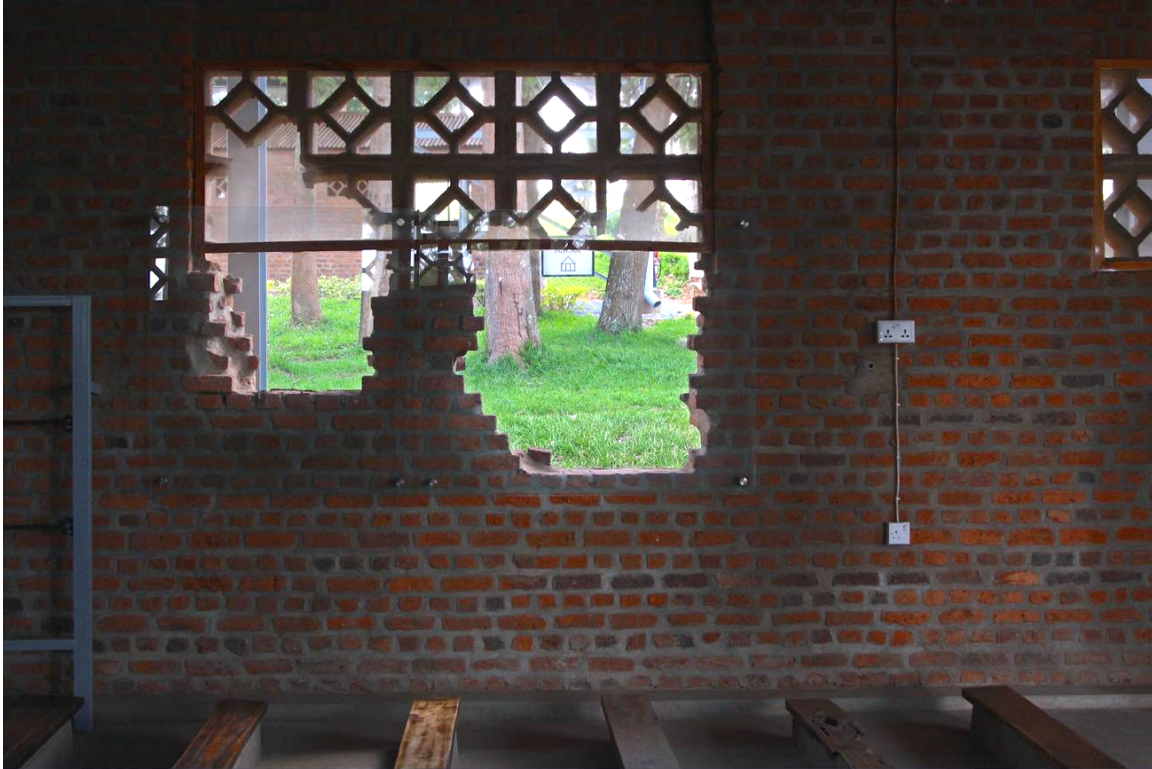
FIGURE 2.19. Preservation work on the church building at Ntarama. A discreet glass panel has been placed in front of the hole to provide maximum visibility of the damage while ensuring that no one can enter the building.
