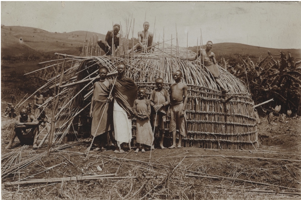
FIGURE 4.4. Construction of a Tutsi dwelling in Rwanda.
