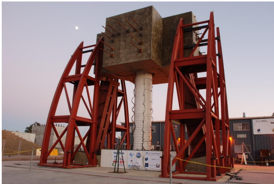
Figure 4.25. Full-Scale Bridge Column Tested Under Seismic Loading at UC San Diego's Large High-Performance Outdoor Shake Table (Schoettler et. al 2012)
