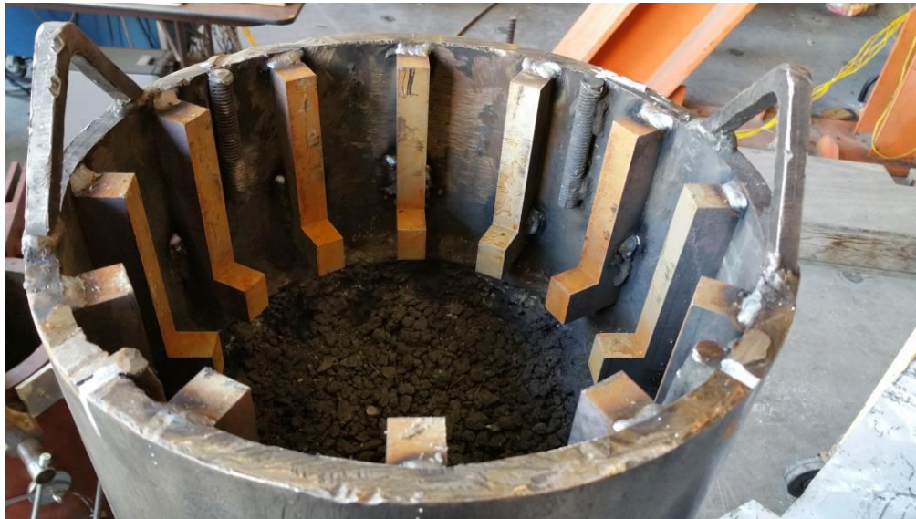
Figure 5.5. L-shaped Brackets Welded Inside the Pipes to Support the Circular End Blocks
