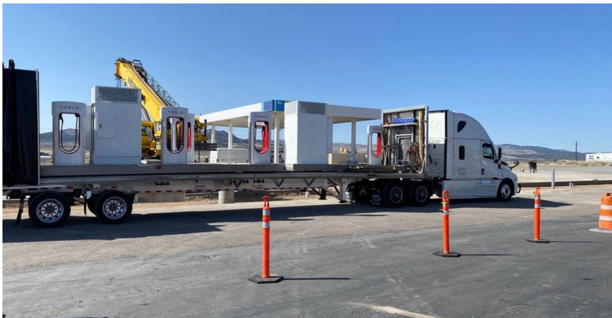
Figure 14: prefabricated charging station modules 5
