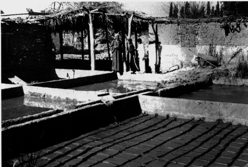
Plate 10.16 Rectangular clay settling basins with water at various stages of evaporation at El Qanatar flowerpot workshop. Note drying sheds in center background; exterior workshop wall appears in left background.
