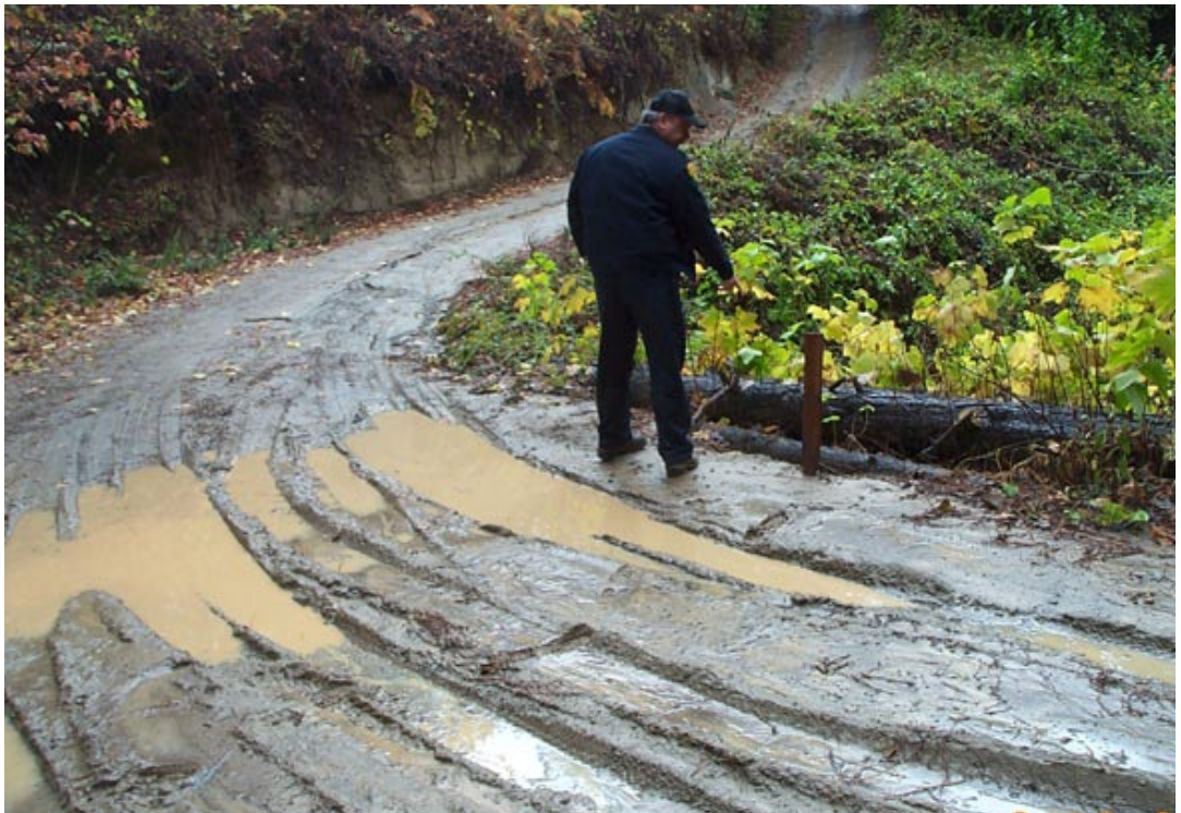
Figure 2. Use of unsurfaced roads in the winter can lead to erosion and sediment delivery to streams. Photo: Courtesy Angela Wilson.
