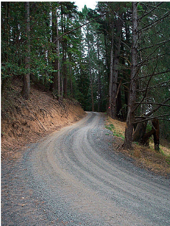
Figure 10. There is a gentle rolling dip in the middle of this picture of an out-sloped road. Photo: Richard Harris.
