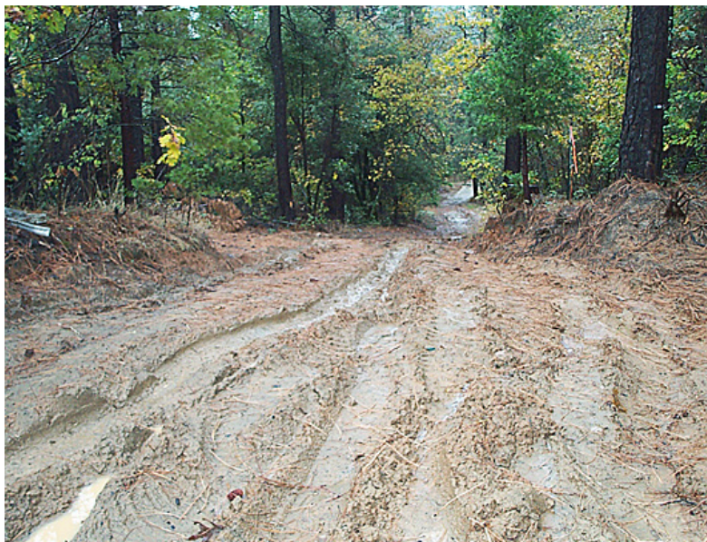
Figure 6. Driving on unsurfaced roads during rainy weather can create ruts and pot-holes that are difficult to repair. Photo: © Angela Wilson; used with permission.
