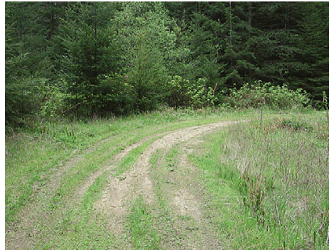
Figure 5. Seasonal-use roads often develop a cover of grass and forbs. This is beneficial for preventing road surface erosion during the winter. Photo: © J. Bawcom; used with permission.
