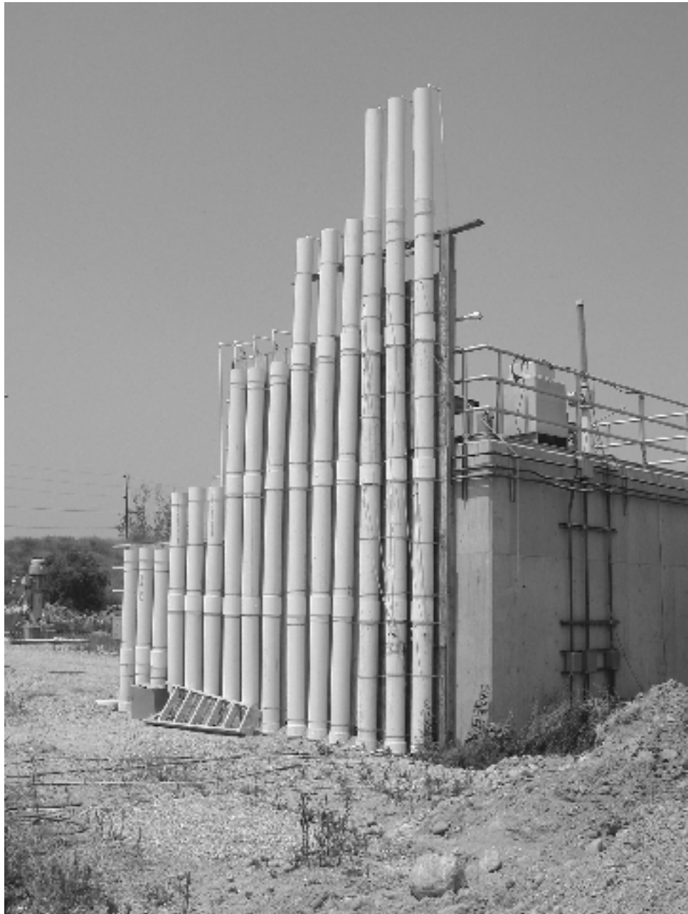
Figure 6. MODIFICATION 2 COLUMNS IN PLACE AT RIX
