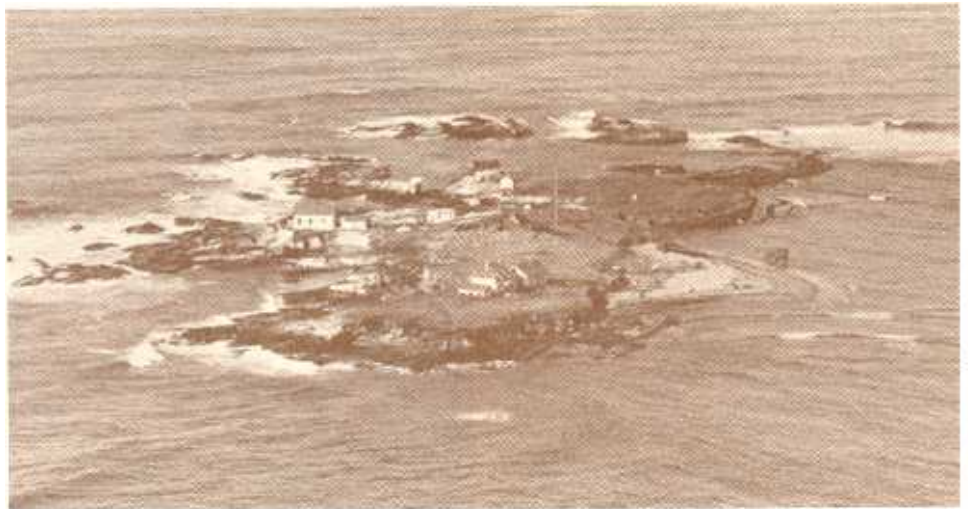
This aerial view shows eight-acre Año Nuevo Island and the former Coast Guard facilities now being renovated with NSF funding. The foghorn building is on the left, and the blockhouse is in the middle of the photo. The lightkeeper's house in the foreground is no longer used.
