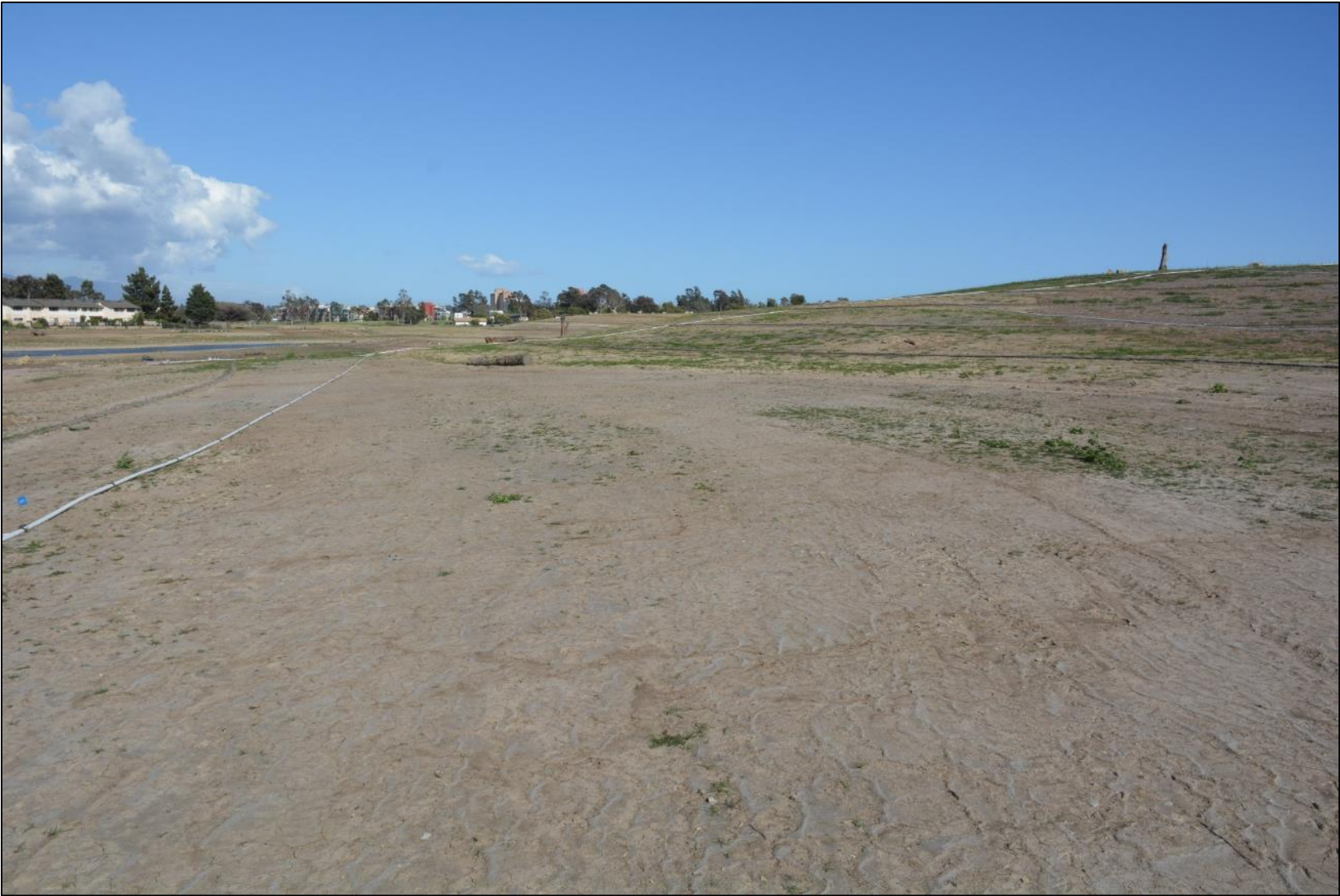
As-built photo - April 16, 2018.
