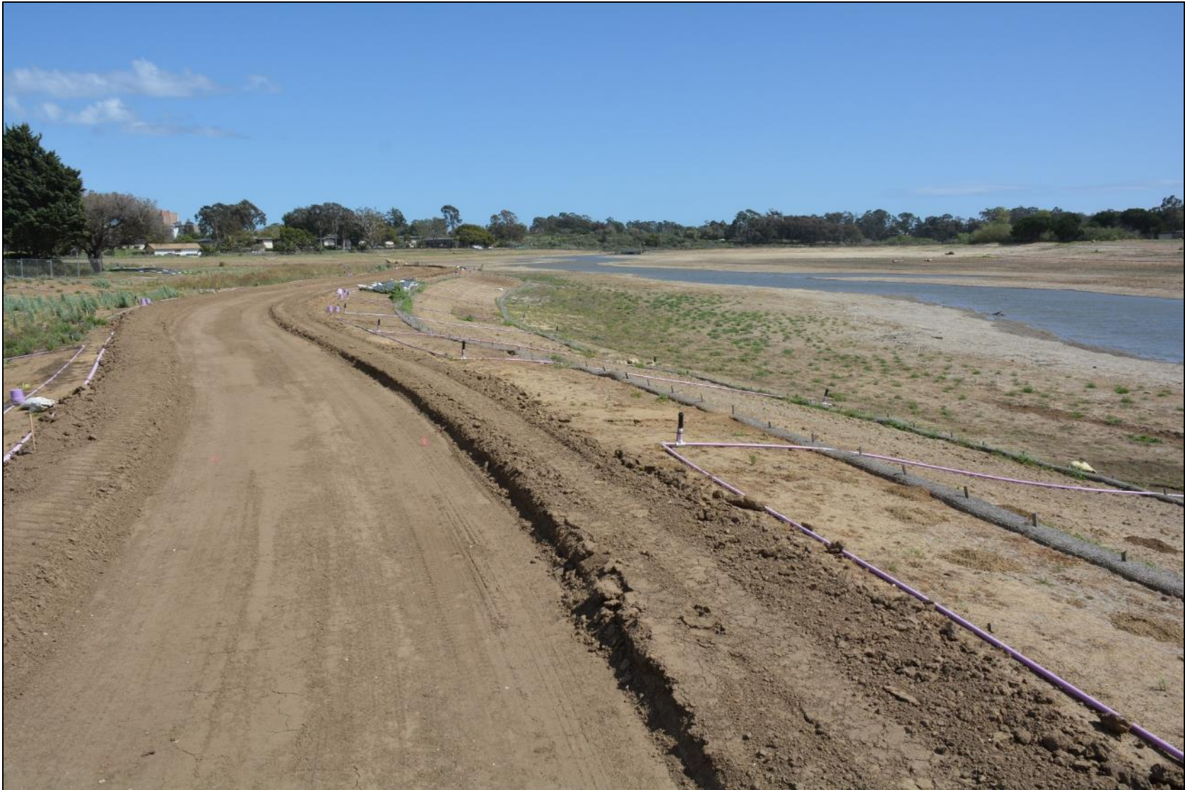
As-built photo - April 16, 2018.
