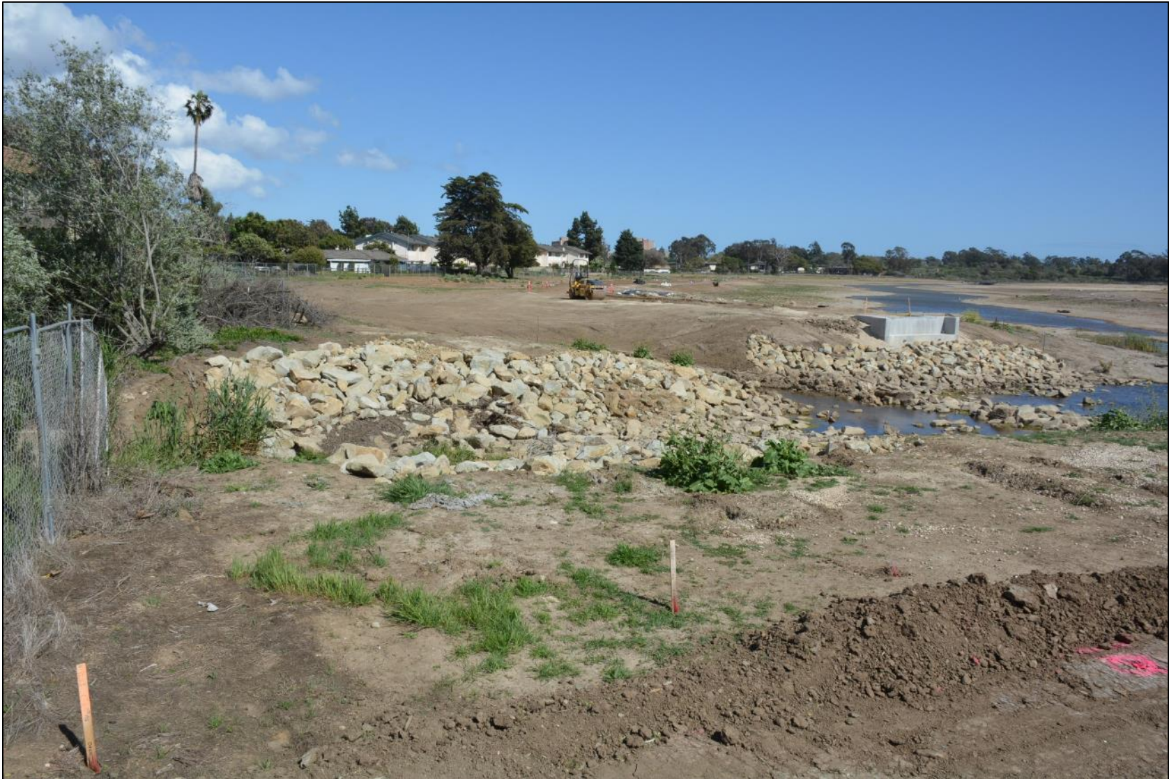
As-built photo - April 16, 2018.
