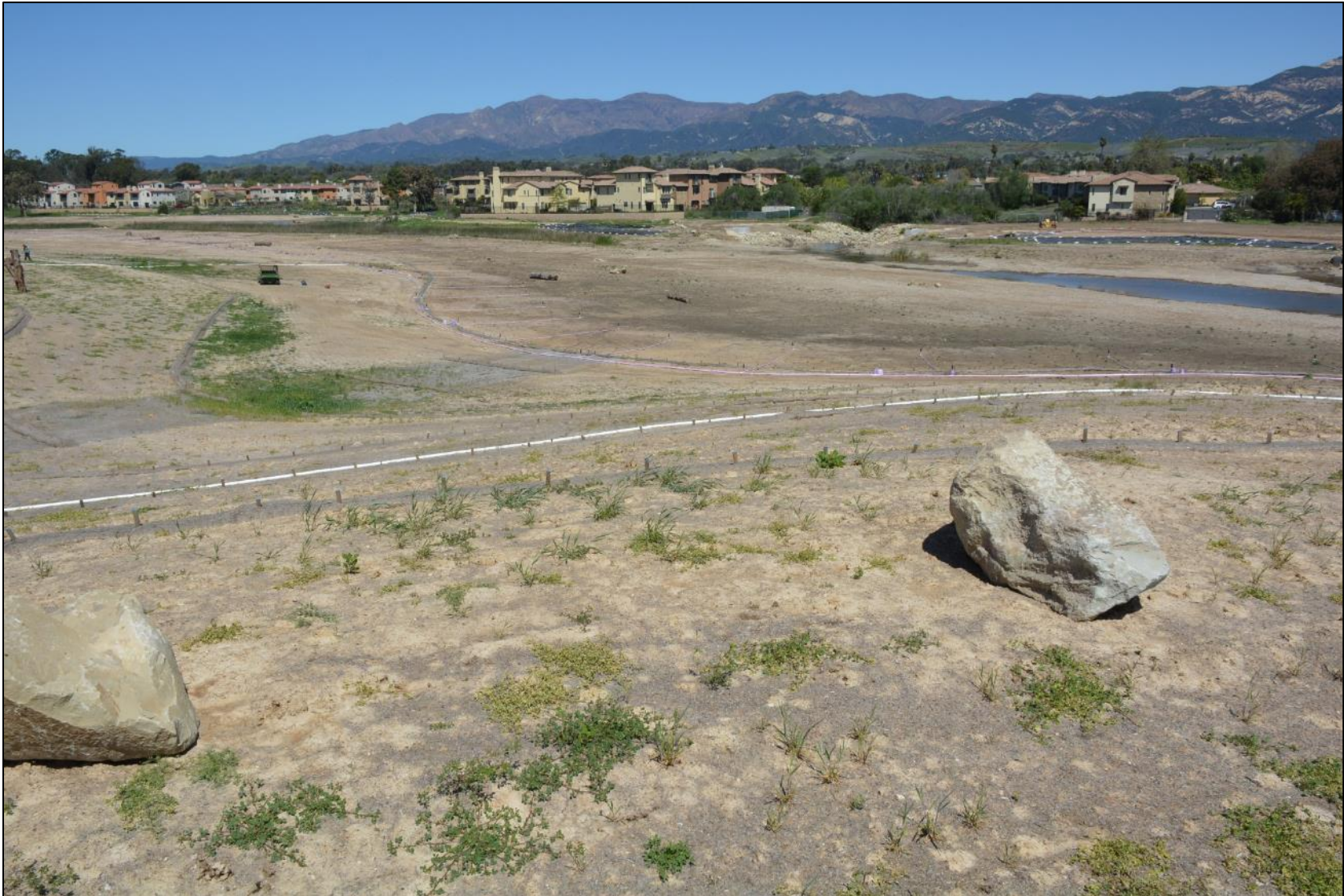
As-built photo - April 17, 2018.
