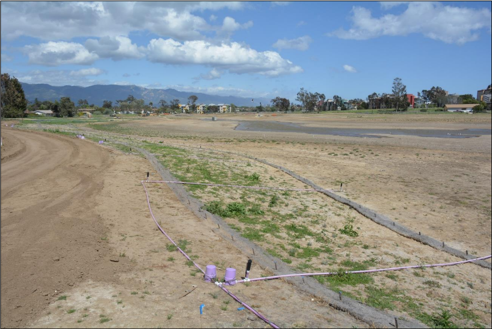
As-built photo - April 16, 2018.
