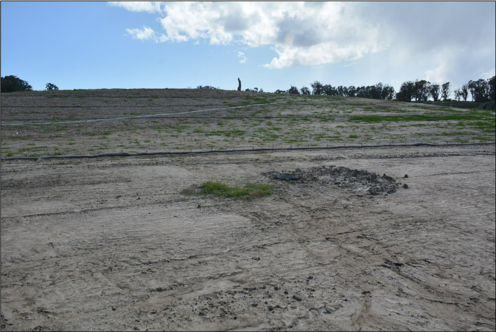
As-built photo - April 16, 2018.
