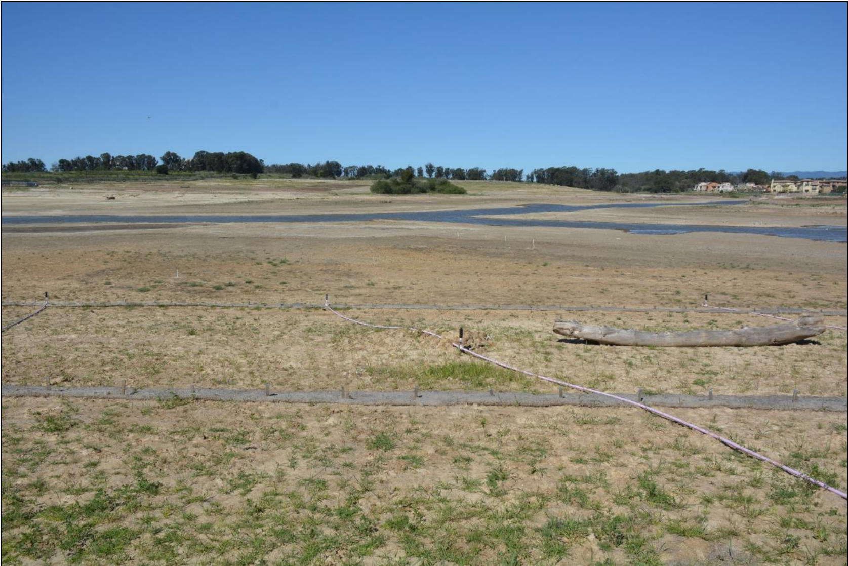
As-built photo - April 17, 2018.
