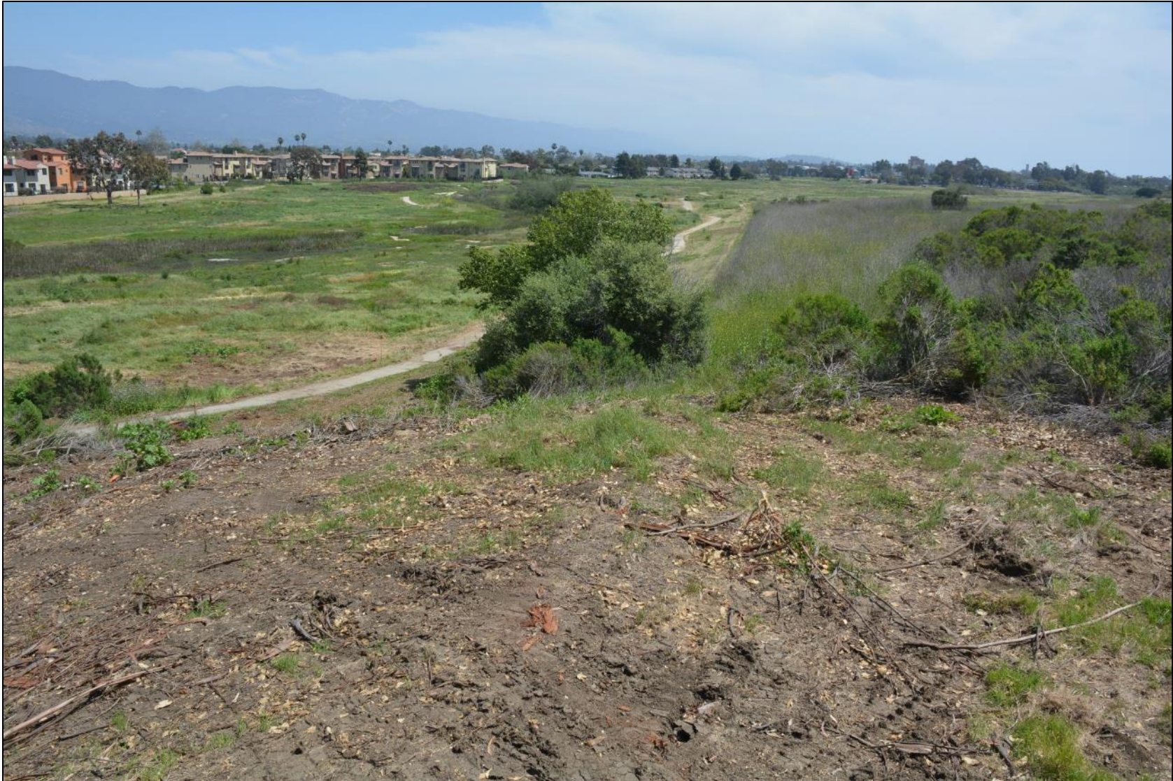
Baseline photo – pre-grading, April 11, 2017.
