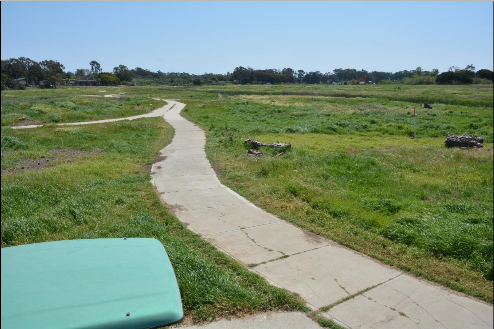
Baseline photo – pre-grading, April 10, 2017.
