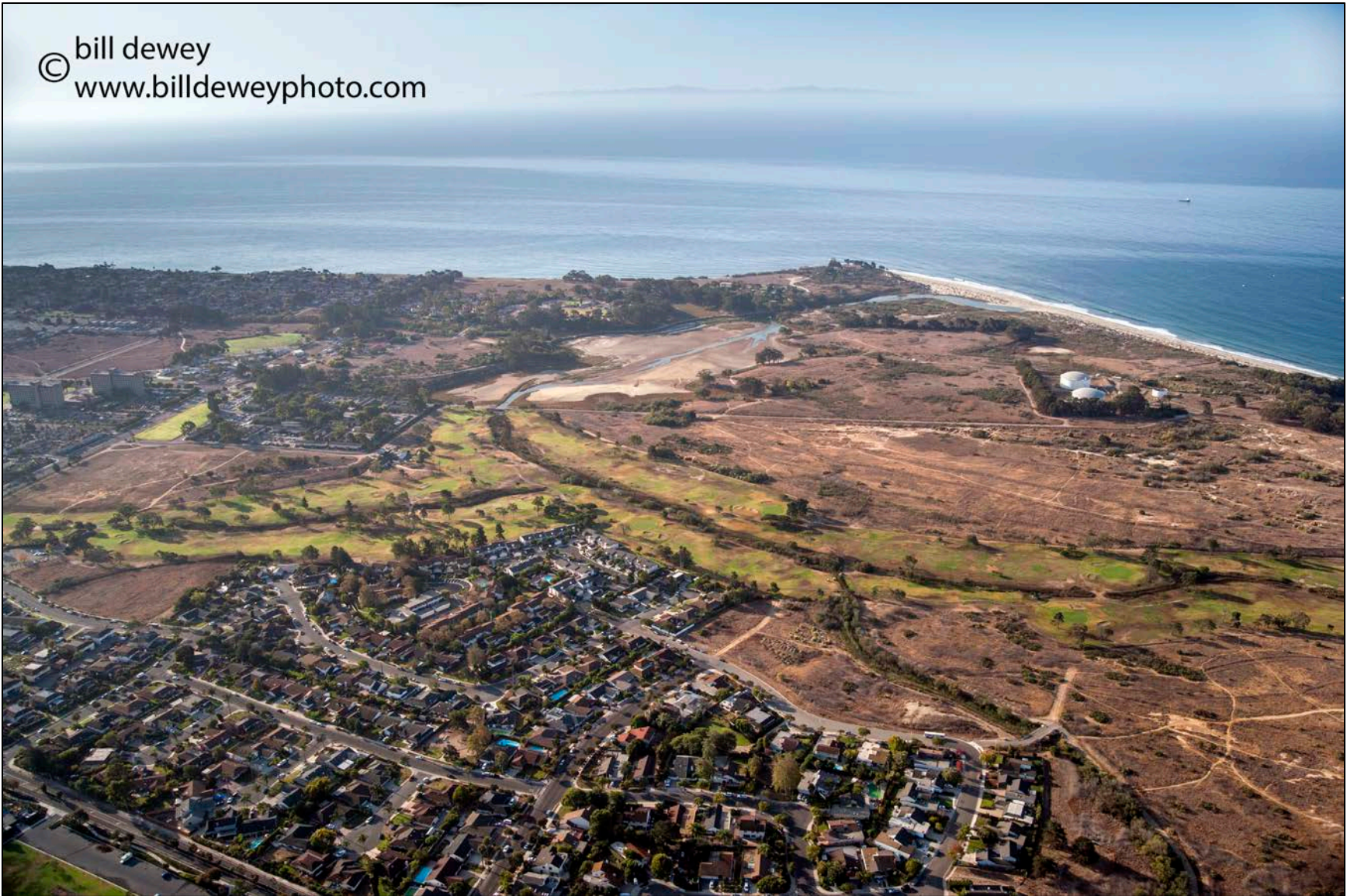
Aerial image of the North Campus Open Space project site, taken by Bill Dewey on October 7, 2009.
