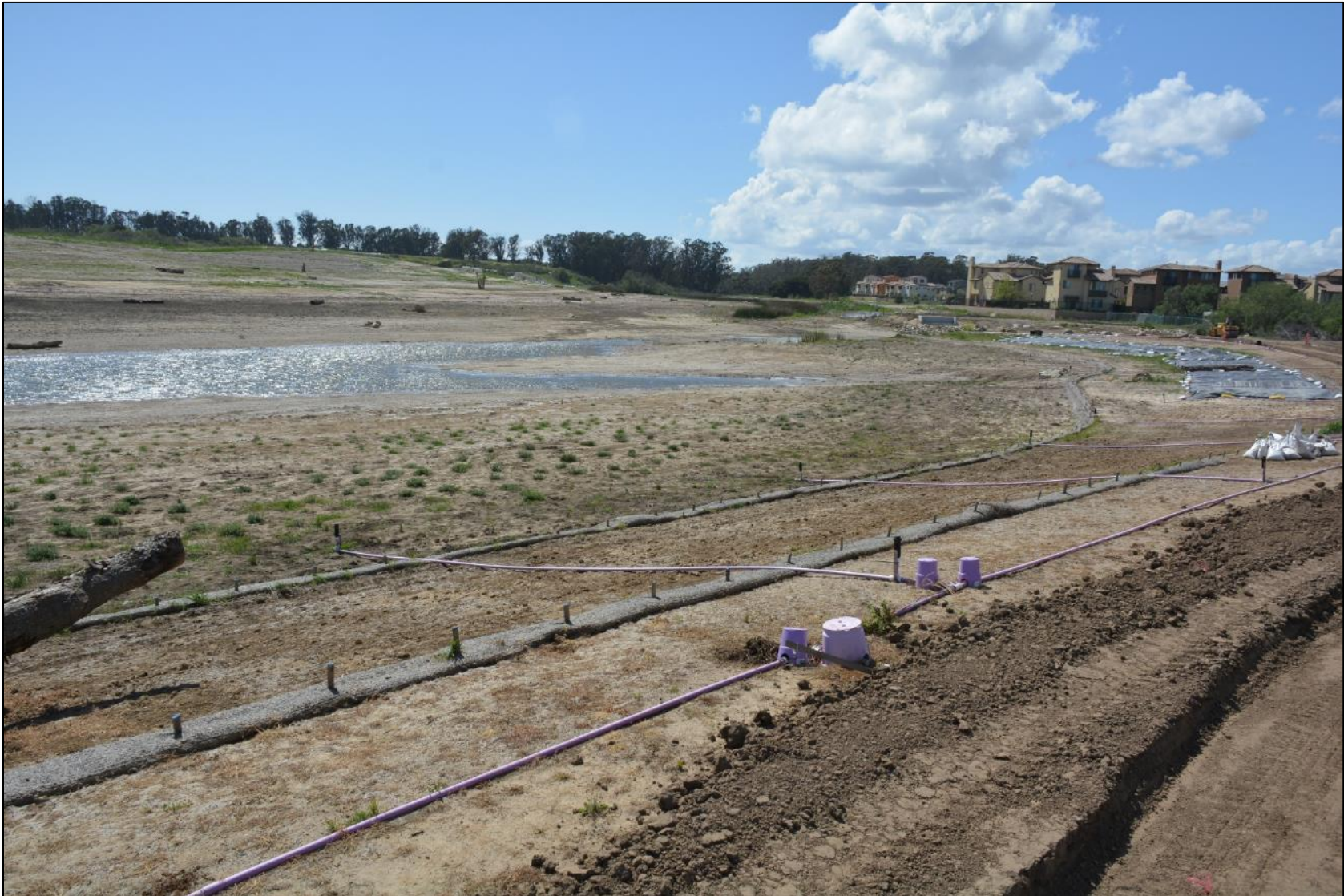
As-built photo - April 16, 2018.
