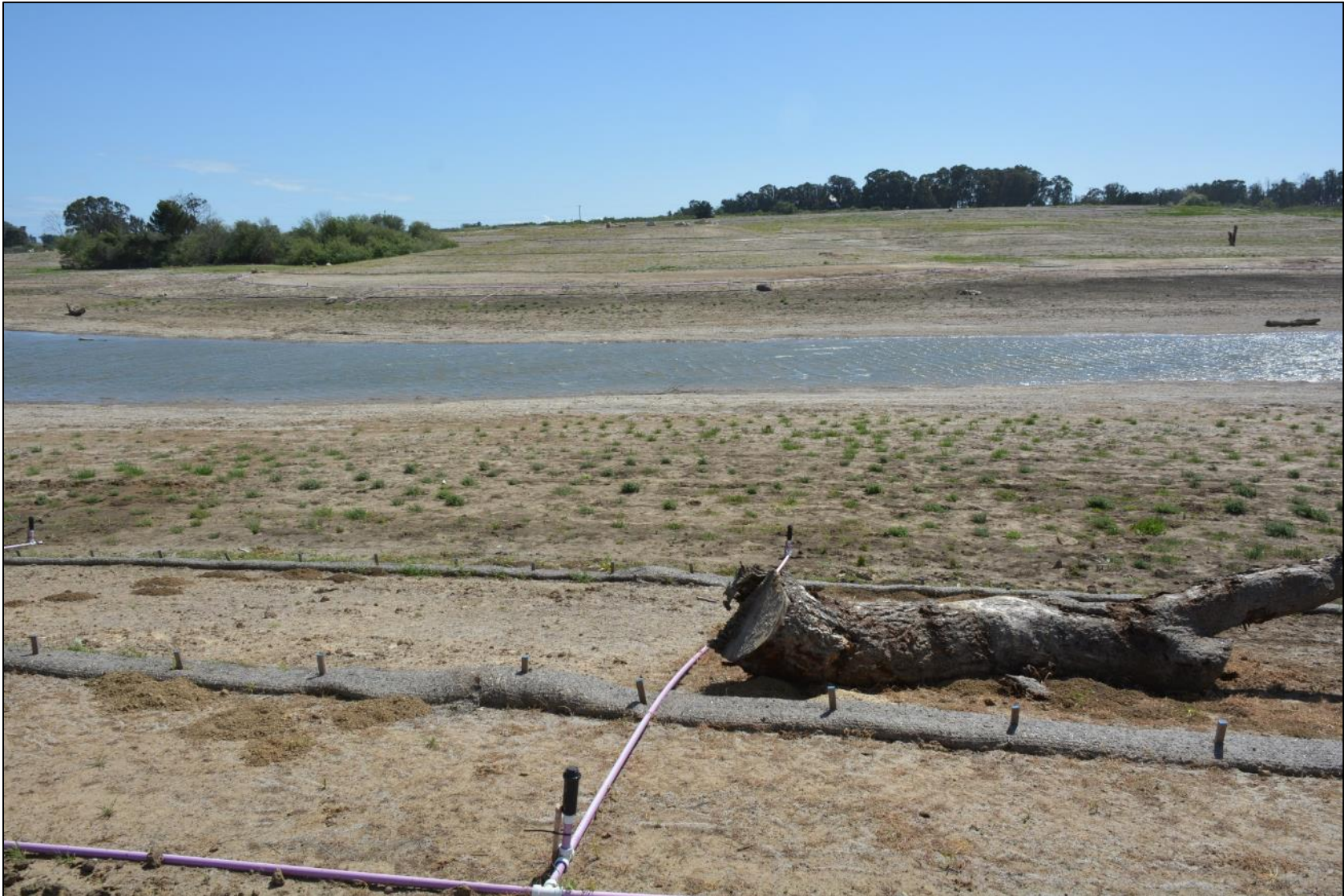
As-built photo - April 16, 2018.
