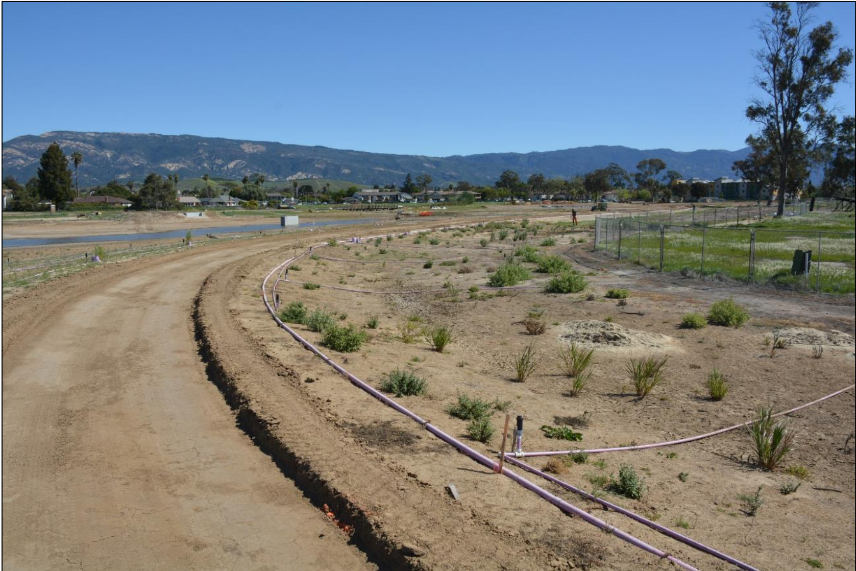
As-built photo - April 16, 2018.
