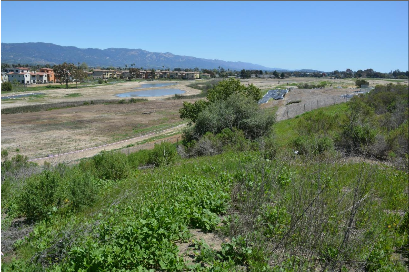
As-built photo - April 17, 2018.
