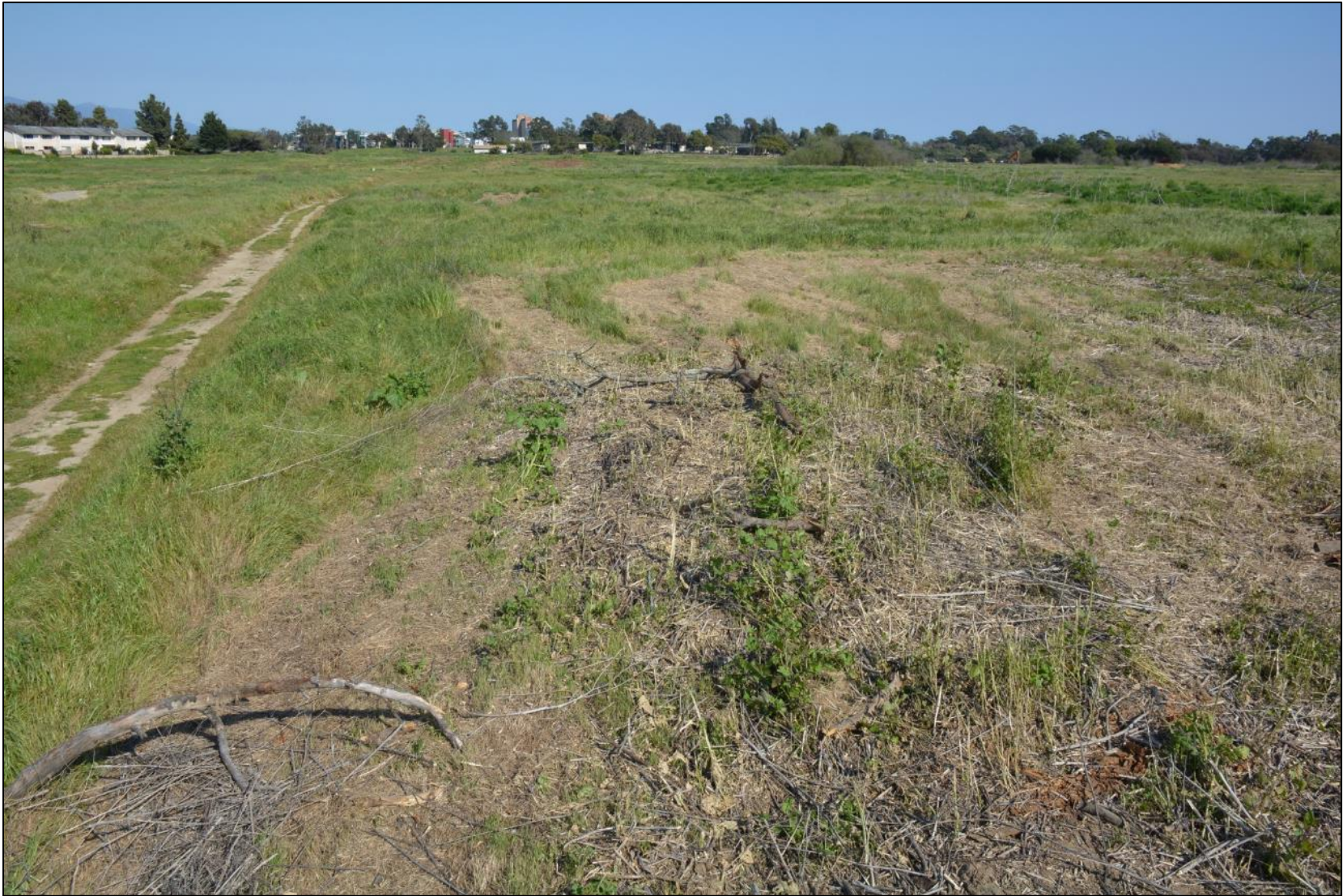
Baseline photo – pre-grading, April 10, 2017.
