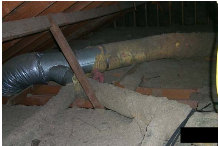
Figure 2. Poorly insulated sheet metal ducts and blown-in insulation in the attic before retrofit
