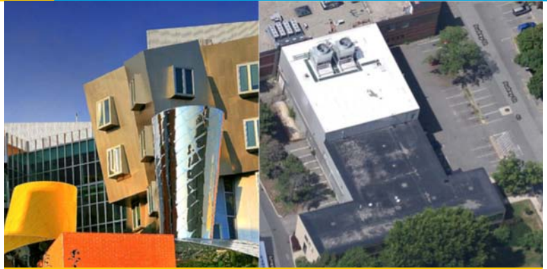
Left: Exterior of the Ray and Maria Stata Center, showing the unconventional geometry of the building envelope. Source: MIT. Right: Overhead view of BW91 Data Center with cooling towers visible on the roof. Source: Google Maps.
