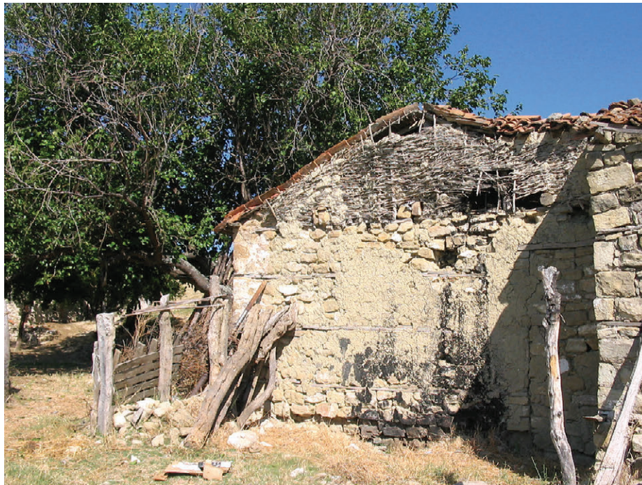
FIGURE 14.2 Ruin of modern wattle-and-daub house in the Lofkënd survey area (photo Jamie Aprile)
