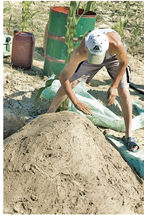
FIGURE 22.6 (continued). Mixing the soil, straw, and water for the making of mud bricks: (c) treading of the mixture; (d) prepared mixture heaped into a pile
