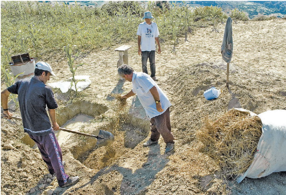
FIGURE 22.6 Mixing the soil, straw, and water for the making of mud bricks: (a) mixing pits with water brought up to the site by donkey; (b) mixing the soil, straw, and water; (c, d) on facing page
