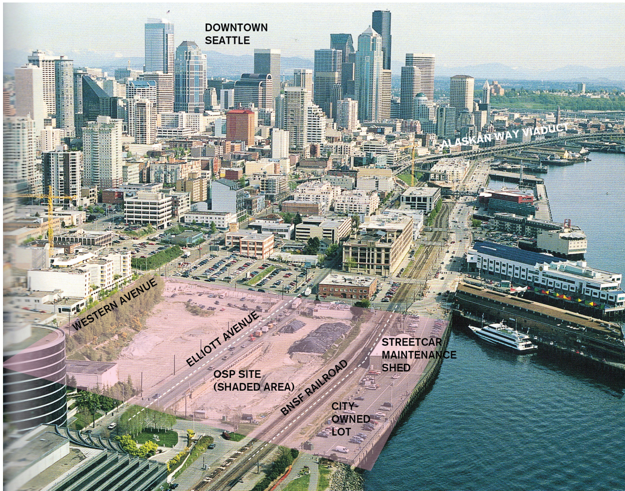
Figure 5.1 Olympic Sculpture Park, Weiss/Manfredi (site diagram) three site parcels separated by road and railroad prior to project implementation (by author)
