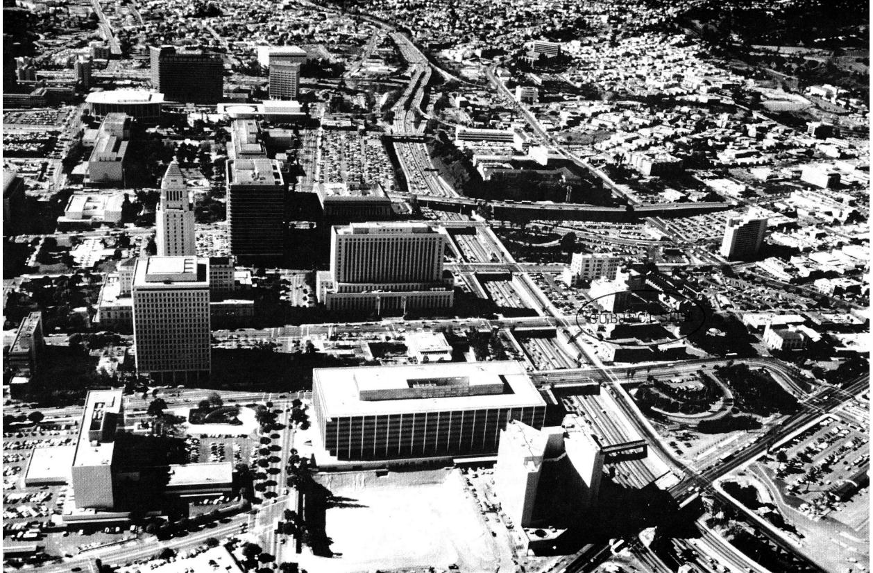
Figure 3.4 Aerial photo of site from southeast from West Coast Gateway Competition Program
