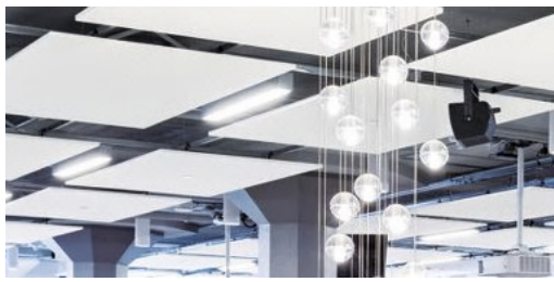
Figure 15: (Left) Example of free-hanging acoustic clouds (image: Armstrong World Industries); (Right) Section schematic of a ceiling with acoustic clouds and ceiling fan in upward and downward blowing directions
