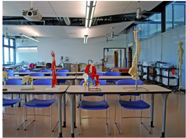
Figure 13: Space using radiant panels: classroom in Lane Community College, Eugene, OR - SRG Partnership Inc. - Image: Lara Swimmer, Steve Wanke
