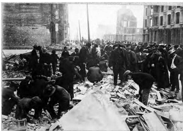
Fig. 64: Photograph titled “San Francisco Earthquake of 1906: Digging for Souvenirs.” Taken by the War Department in April 1906. Courtesy of the National Archives and Records Administration/Wikimedia Commons.
