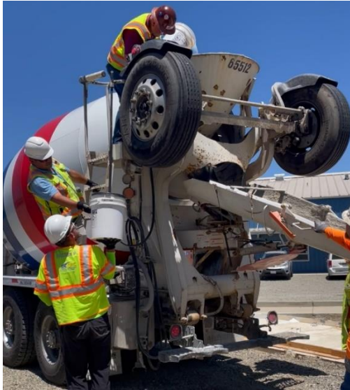
244 Figure 2. Adding the CNC suspension to the ready-mix truck from the hopper at the construction 245 site
