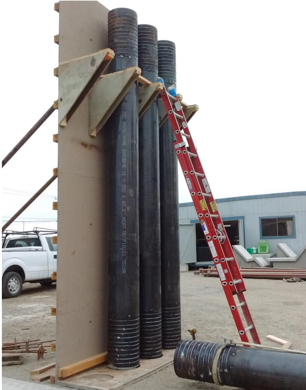
Figure 5.5 Column casting setup
