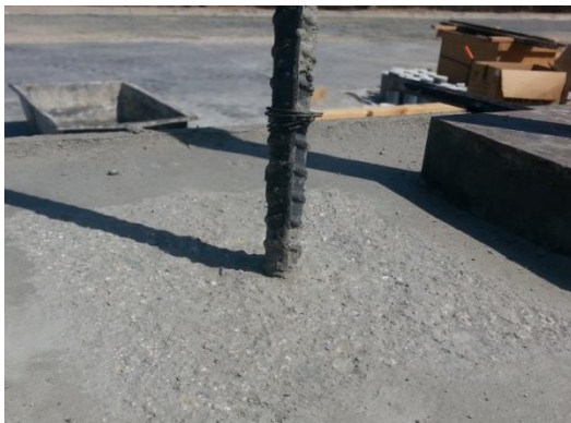
(a) Central bar pre-installed in foundation
