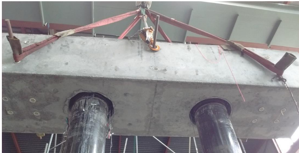
Figure 5.9 Cap beam erection
