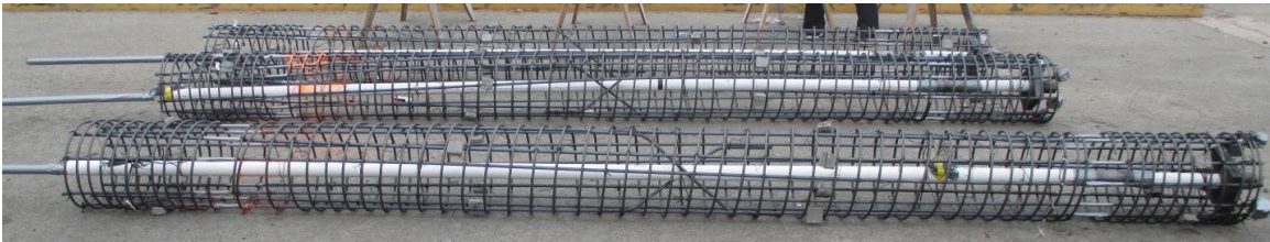
(c) Column reinforcement cages
