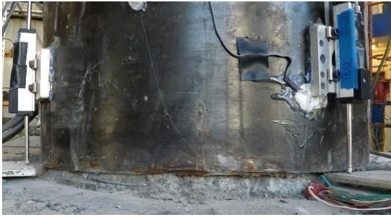
(a) South column interface, North face, \Delta=5.4\%
