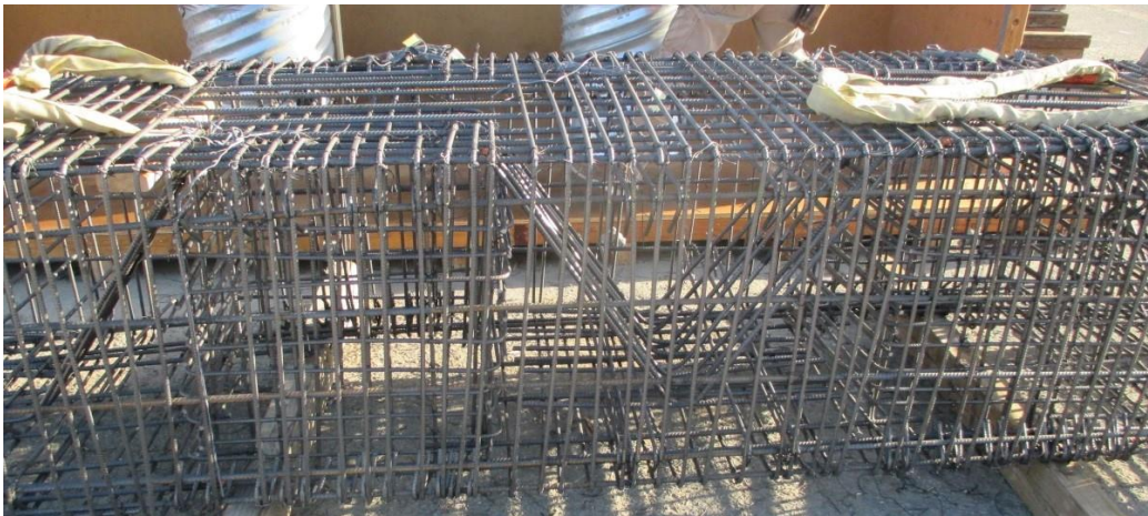
(b) Socket reinforcement detail in cap beam
