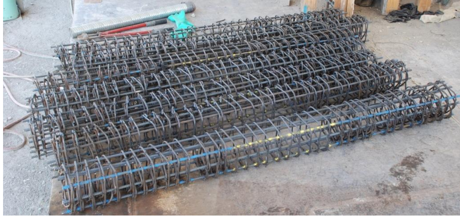
(a) Gravity column perimeter reinforcement cage
