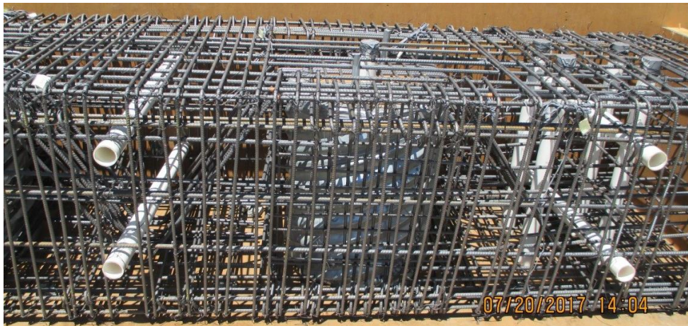
(c) Completed reinforcement cage, cap beam
