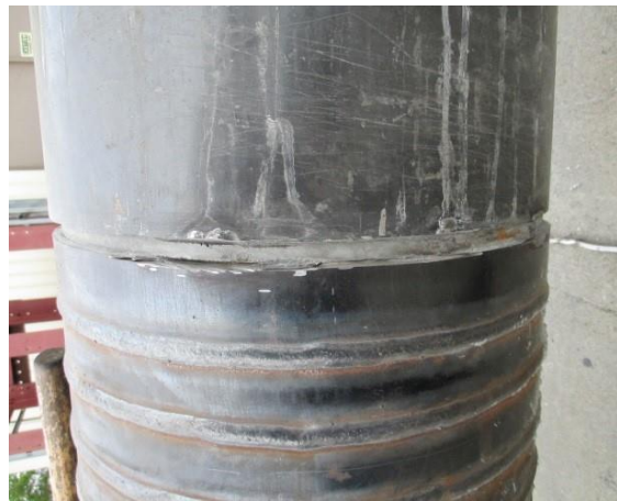
(b) Shell strip removed
