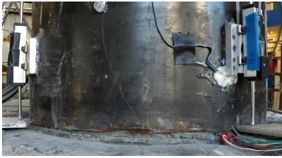
(a) South column interface, North face, \Delta=3.2\%
