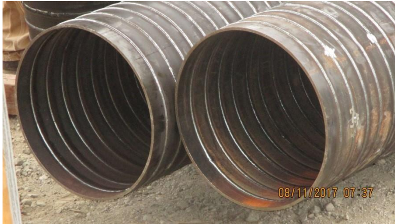
(b) Weld beads at column ends
