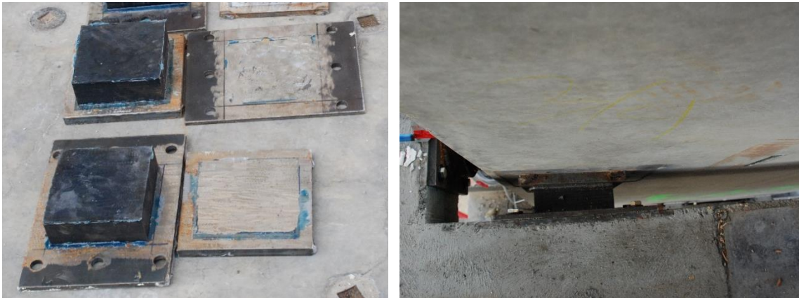
Figure 3.18 Elastomeric bearings
