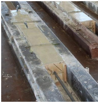
(b) Columns with fresh poured concrete
