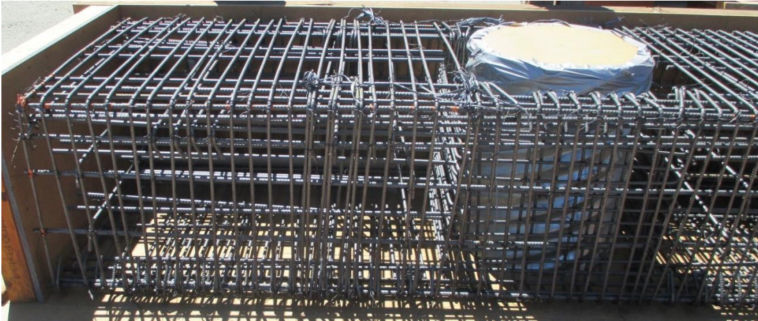
(a) Socket detail in foundation
