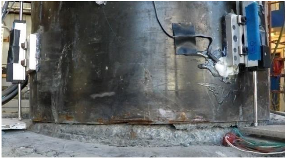
(a) South column interface, North face, \Delta=7.2\%
