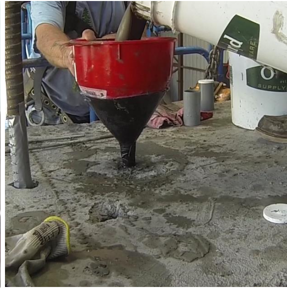
(b) Cap-beam socket grouting
