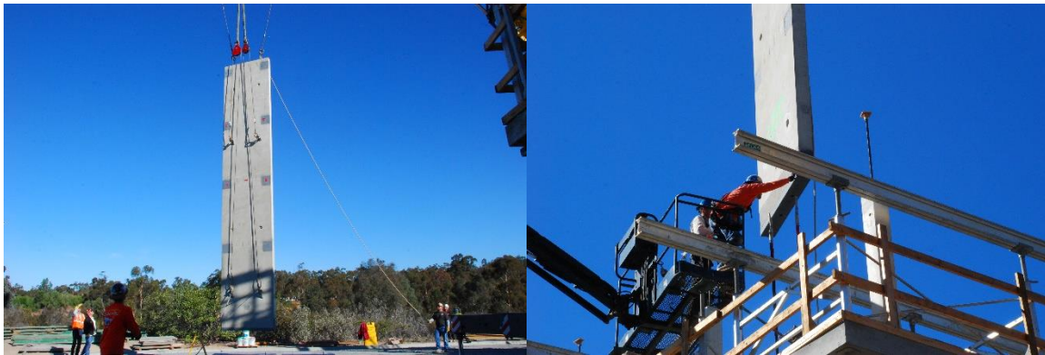
(a) North wall being lifted
