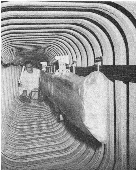
Fig. 15 Installed quadrant cryopanel.
